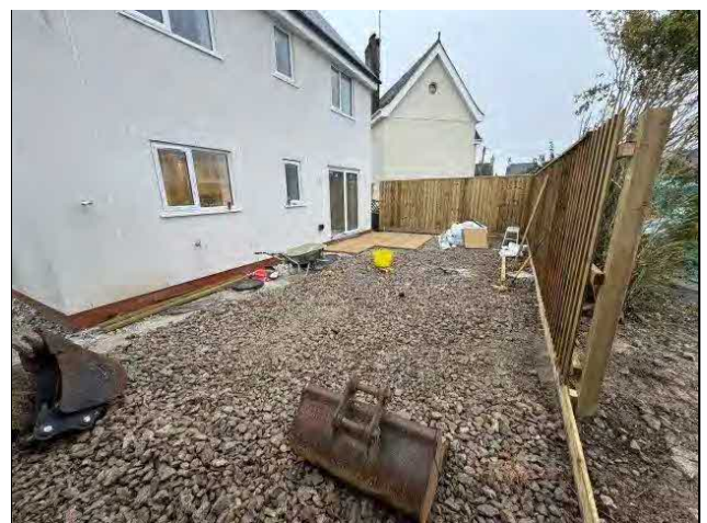
Plate 16: View showing aggregate hardcore capping soils in garden area.
