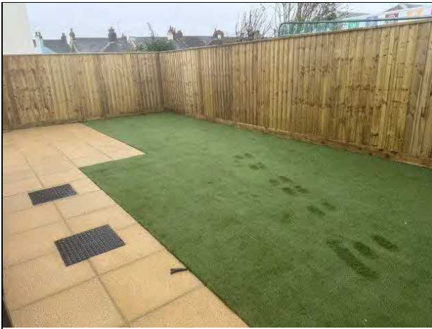
Plate 17: View showing completed garden area with paving.
