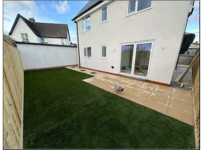
Plate 18: View showing completed garden area with paving.
