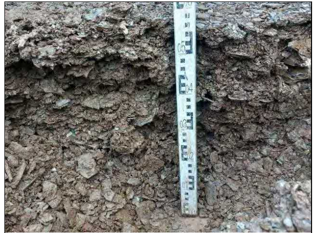
Plate 08: View showing 550mm capping thickness in TP0'
