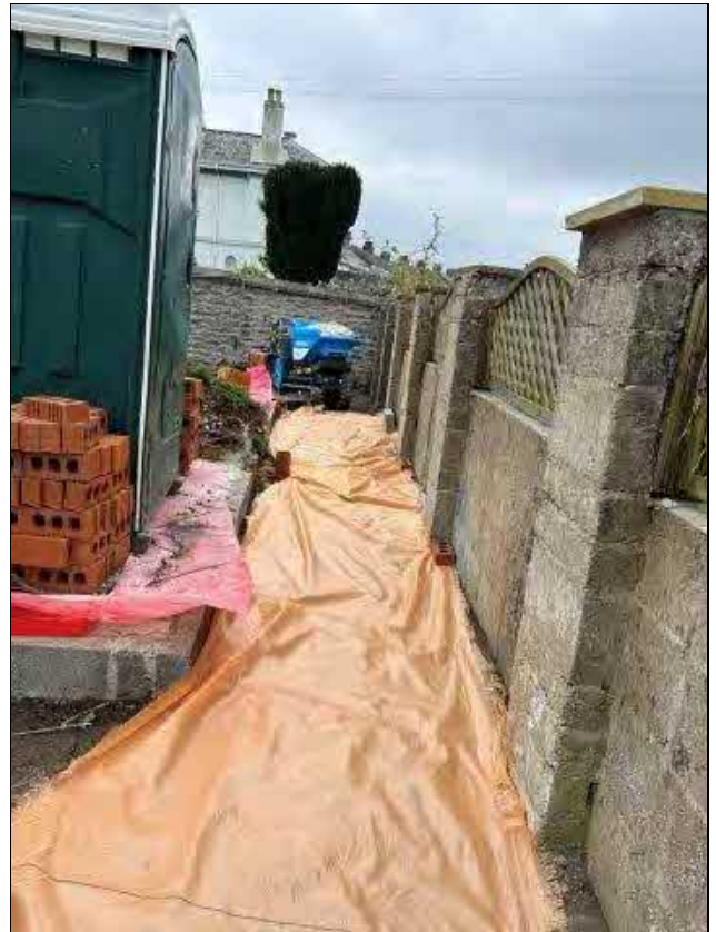
Plate 04: View showing membrane laid over rear patio area.
