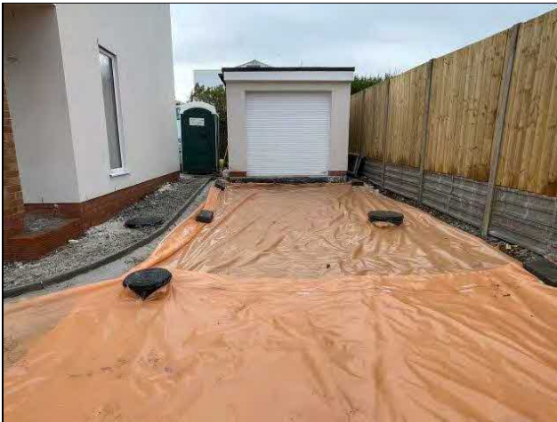
Plate 13: View showing additional separation membrane placed in driveway area over hardcore.
