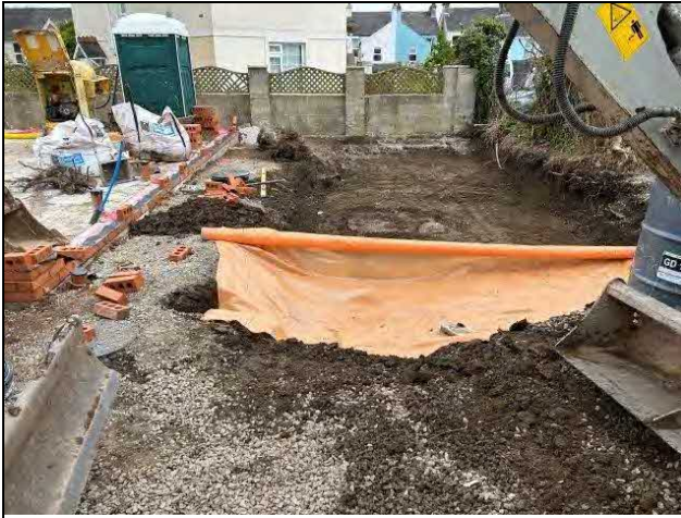
Plate 01: View showing membrane being laid over contaminated soils in garden area.
