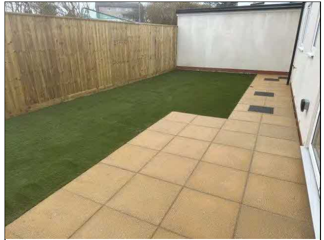
Plate 18: View showing completed garden area with paving.
