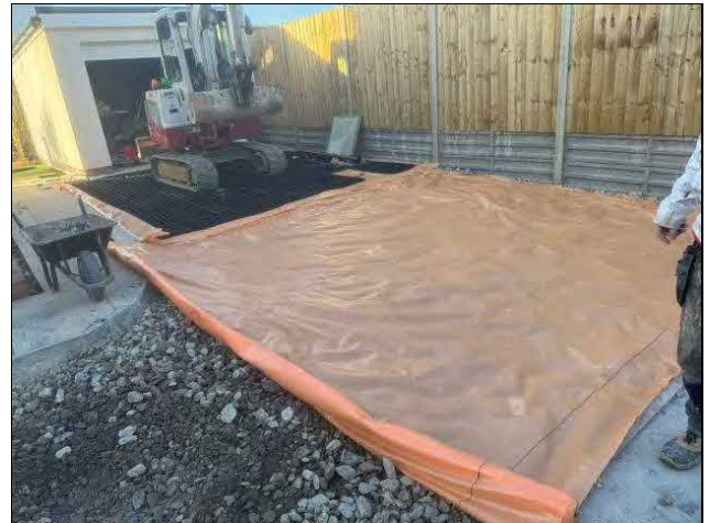
Plate 14: View showing driveway preparation.
