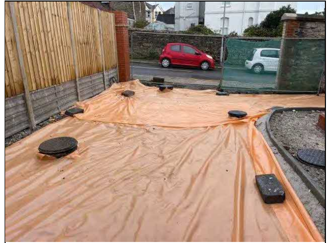
Plate 02: View showing membrane laid over driveway area.
