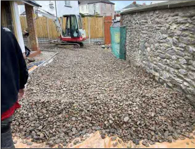
Plate 05: View showing aggregate hardcore | membrane in driveway area.
