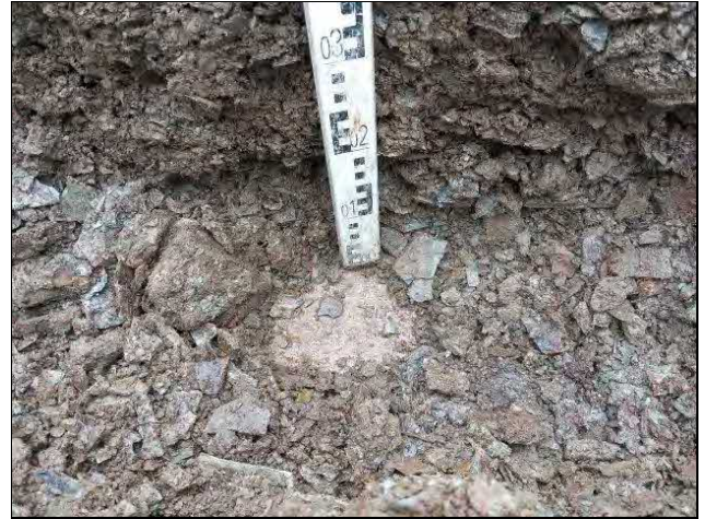
Plate 12: View showing separation membrane at b TP02.
