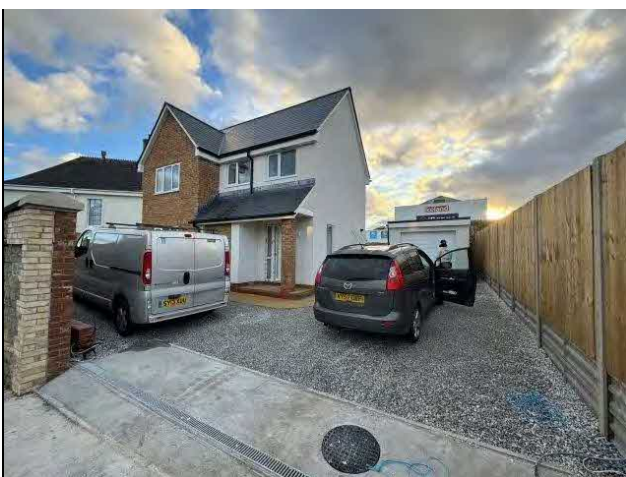
Plate 15: View showing completed driveway.
