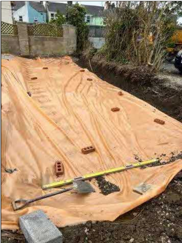
Plate 03: View showing membrane laid over contaminated soils in garden area.
