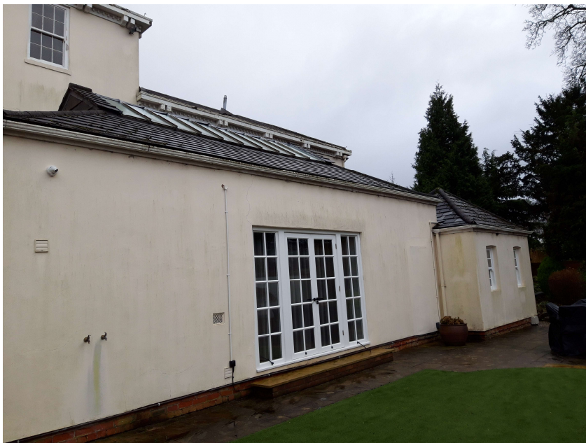
Photo 3 – Location of roof for proposed solar panels
