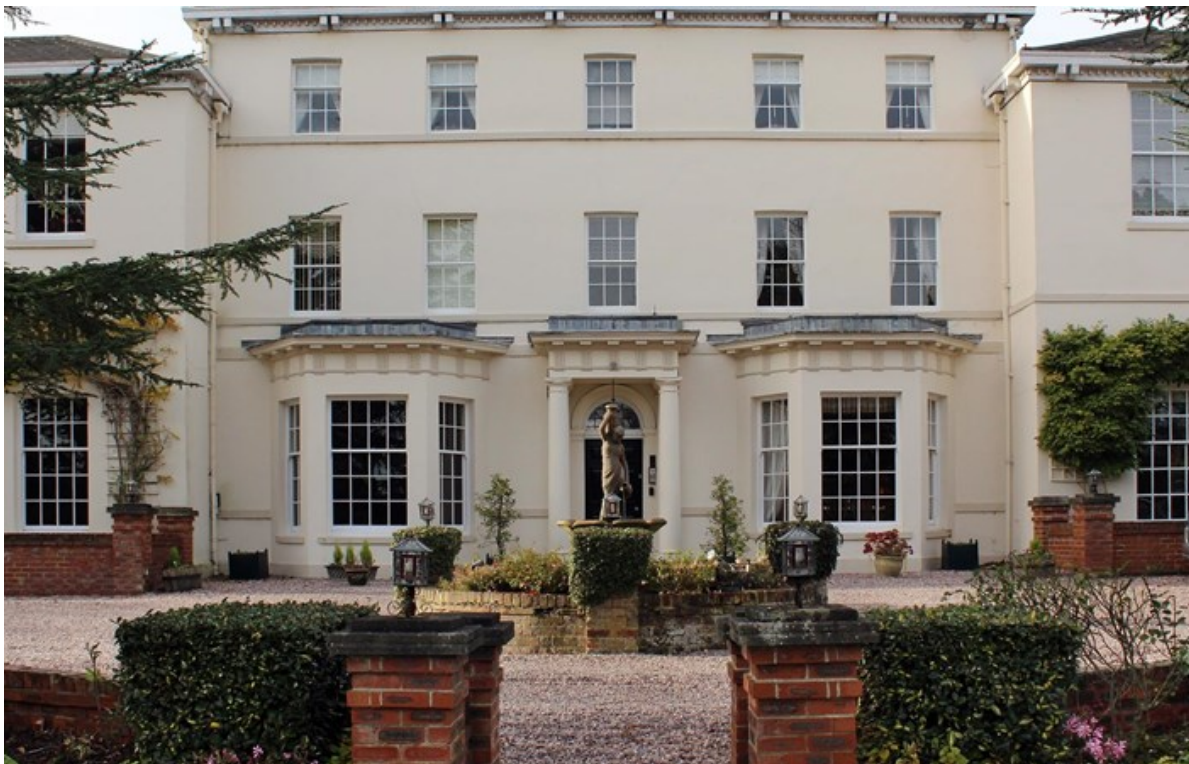
Photo 1 – View of front of Swanland Hall.
