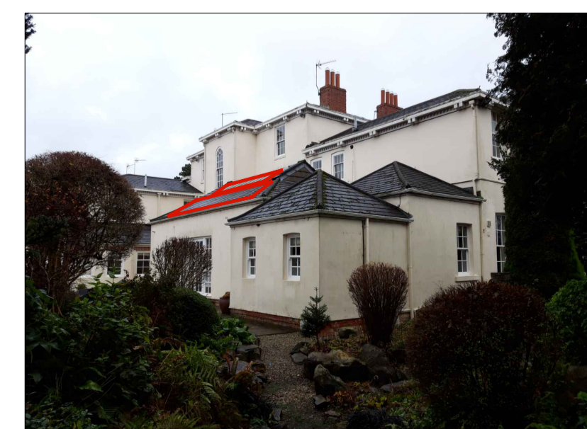
Photo of Elevation with Solar Panels
