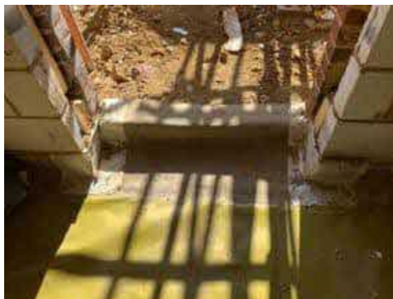
Plot 45 sealed door threshold detail using SAGM.
