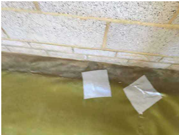
Patch repairs using SAGM to damaged membrane.
