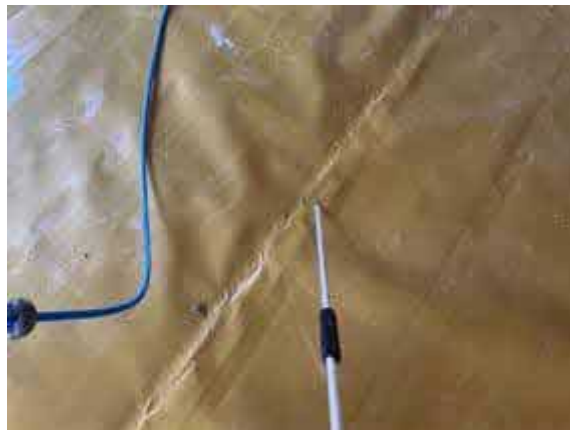
Plot 40. Air lance integrity conducted upon all welded membrane lap joints.
