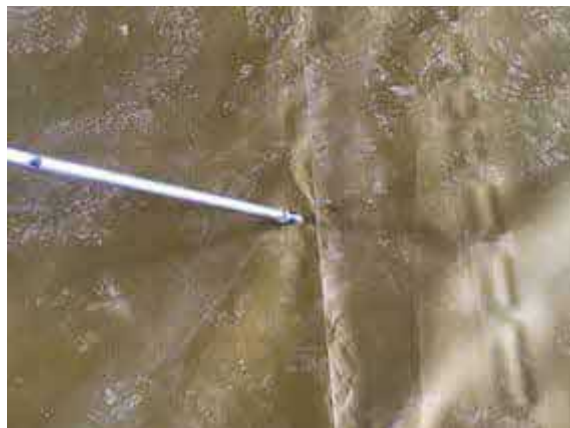
Plot 7 air lancing all welded membrane laps.
