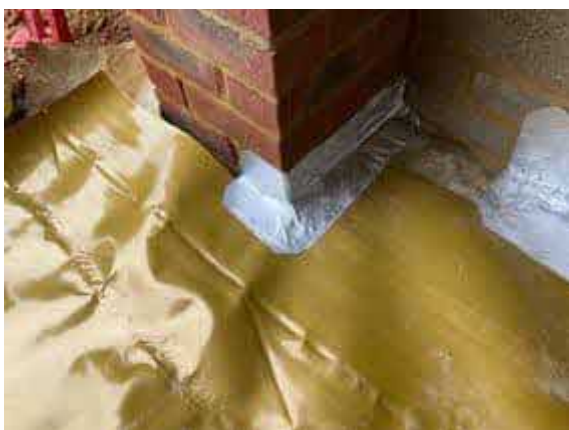
Plot 35 garage. Corner detailing sealed using SAGM.
