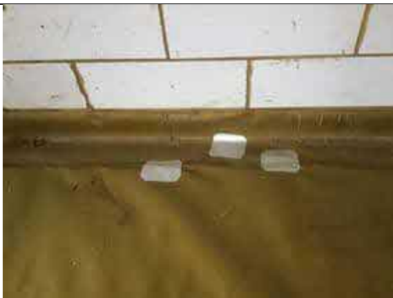
Patch repairs using SAGM to plot 36.
