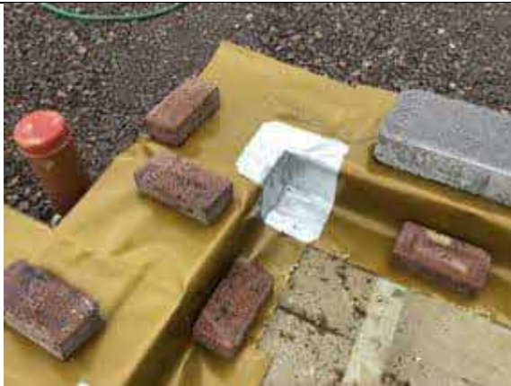
Plot 73 typical corner seal using SAGM.
