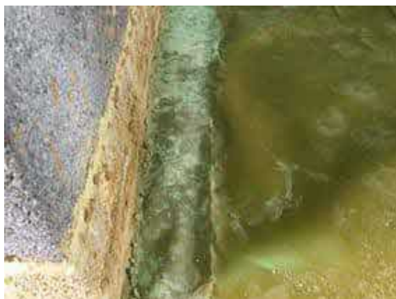
Overview to the perimeter membrane welded to the infill membrane.
