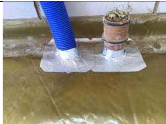
Plot 75 typical double pipe penetration seal using SAGM.
