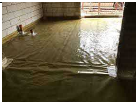
Overview of installed membrane to apartment block C.
