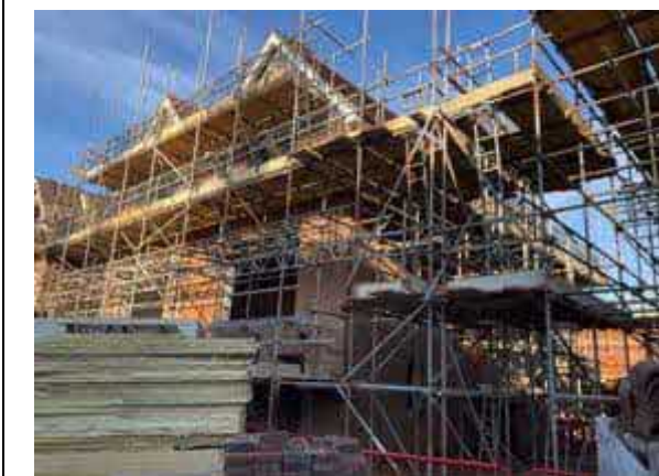
Plot 40 overview of where the installation took place.
