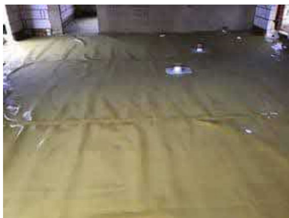
Overview of installed membrane to plot 41.
