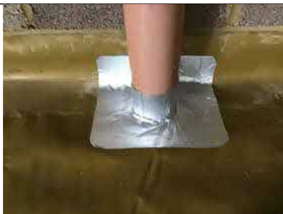
Typical pipe penetration seal using SAGM.
