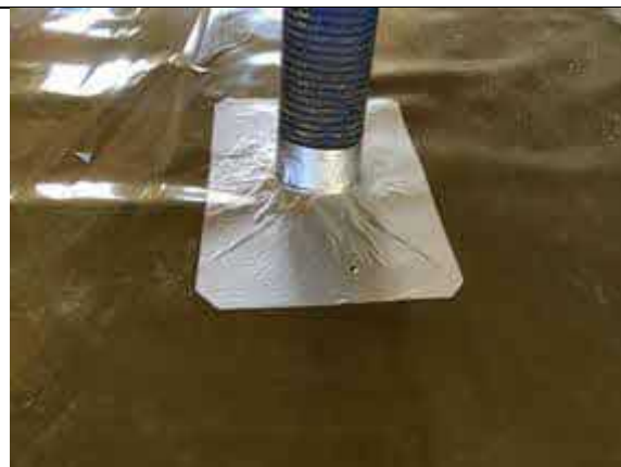
Plot 4 typical pipe penetration seal using SAGM.
