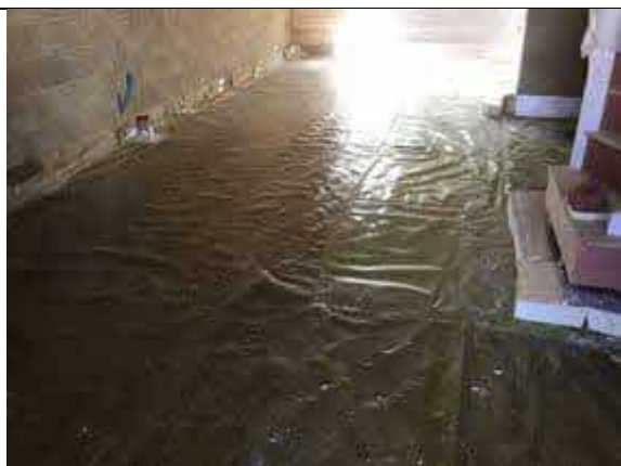
Overview of installed membrane to plot 65.
