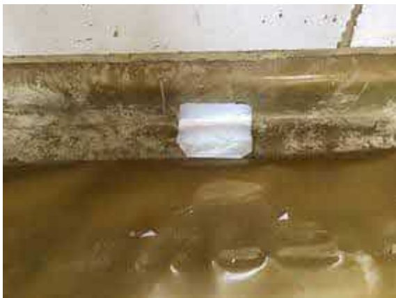
Plot 7 patch repair using SAGM.
