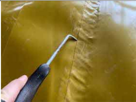
Plot 74. Pick test upon hand welded membrane lap joint.
