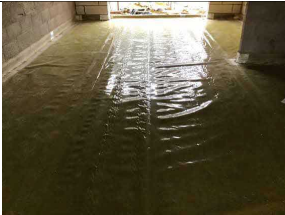
Hand welded membrane lap in plot 51.
