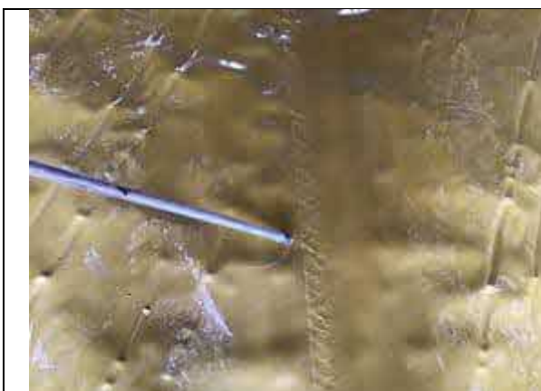
Plot 27 air lancing all weld laps.
