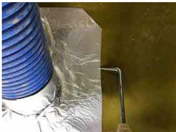
Pick testing all SAGM detailing in plot 50.
