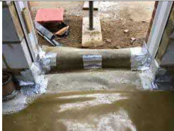
Door threshold seal using SAGM.
