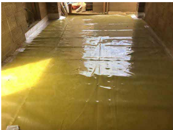
Overview of installed membrane to the garage, as an infill to plot 71.
