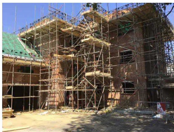
Overview of Apartment Block H. Plots 54-62.
