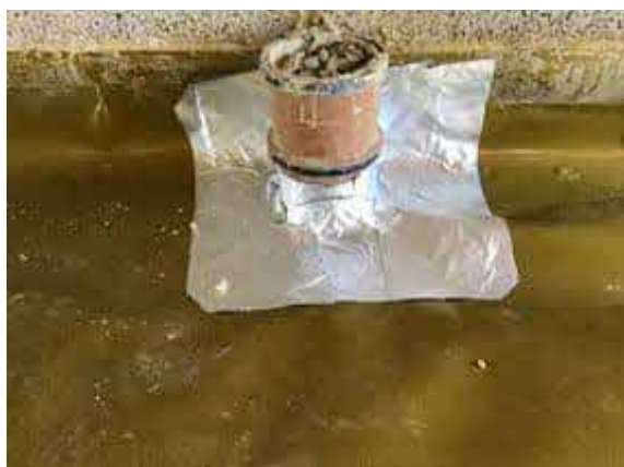
Plot 2 typical pipe penetration seal using SAGM.
