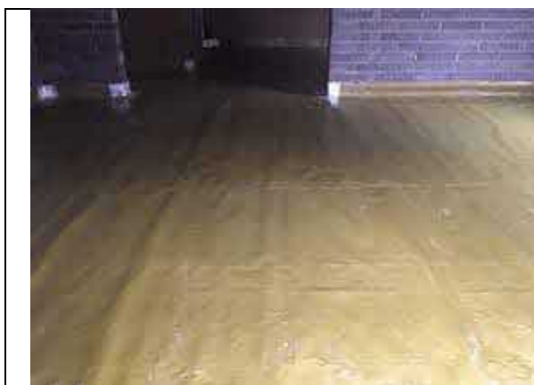
Overview of installed membrane to apartment block C.
