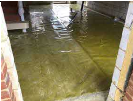
Overview of installed membrane to plot 50.
