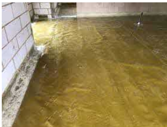
Plot 76 overview of installed membrane.
