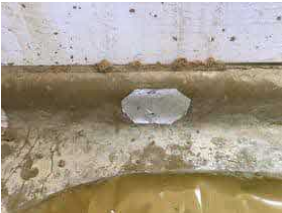
Plot 32 patch repair to damaged membrane caused by follow on trades and repaired using SAGM.
