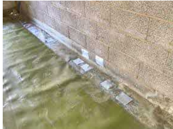
Patch repairs to damaged perimeter membrane using SAGM to plot 67.
