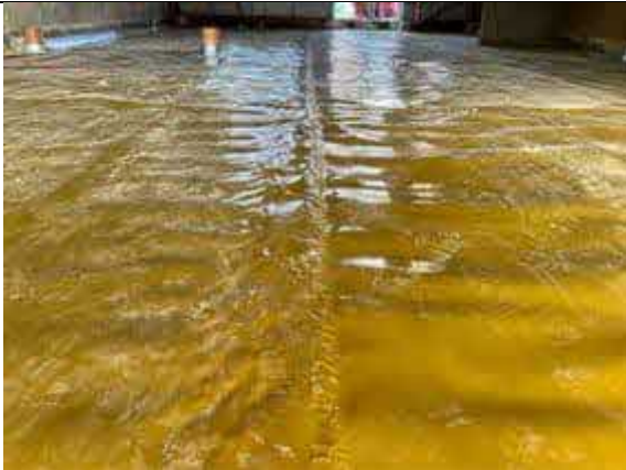
Plot 29 - Successfully hand welded membrane lap joint.
