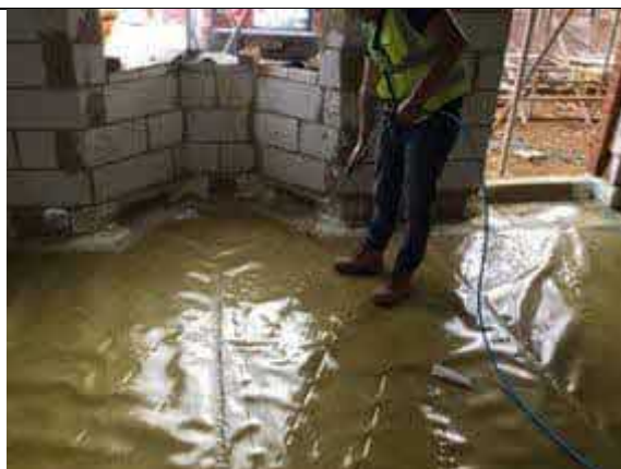
Air lance testing to Plot 10 lap joints.
