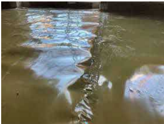
Plot 40. Hand welded membrane lap joint.
