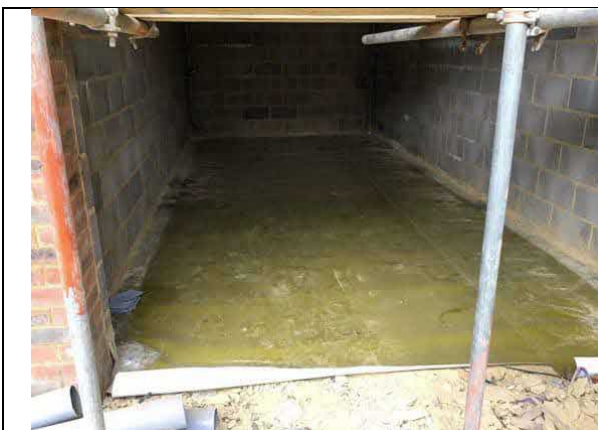
Overview of installed membrane in garage plot 63.
