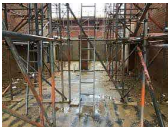
Scaffolding in place in all garages.
