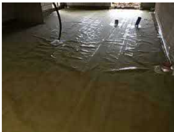
Overview of installed membrane to plot 39.
