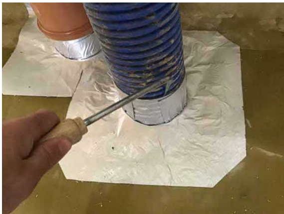
Pick testing all SAGM detailing in plot 52.
