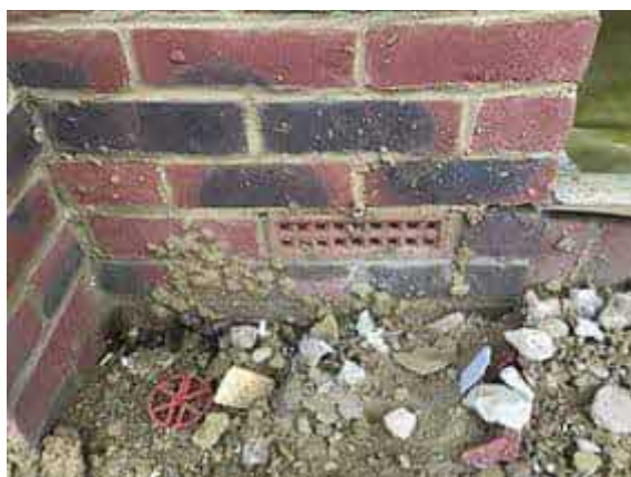
Air brick in place to plot 41.
