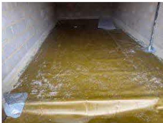
Overview of Visqueen HC Blok infill installation to Plot 32 FOG Unit Garage.
