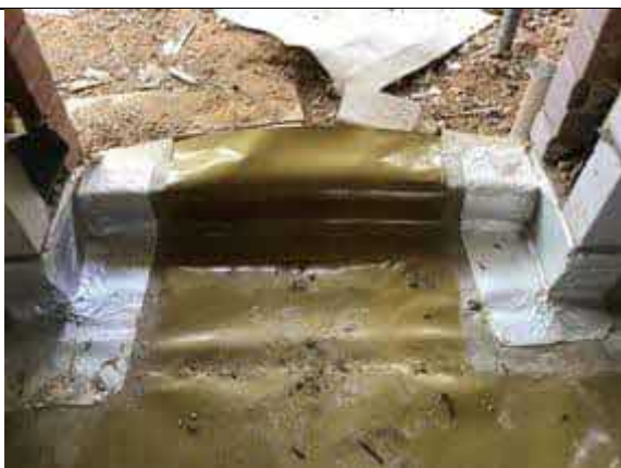
Sealed door threshold using SAGM.
