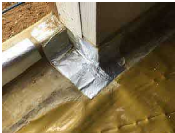
Sealed corner detail using SAGM.
