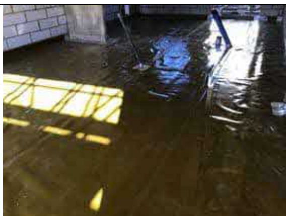
Plot 2 overview of installed membrane.
