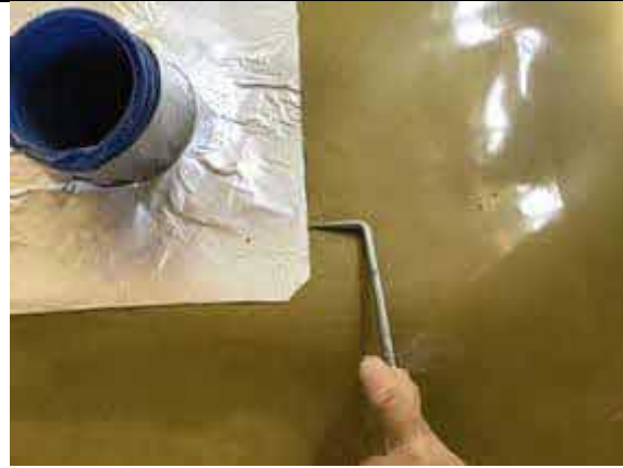
Pick testing all SAGM detailing to plot 67.
