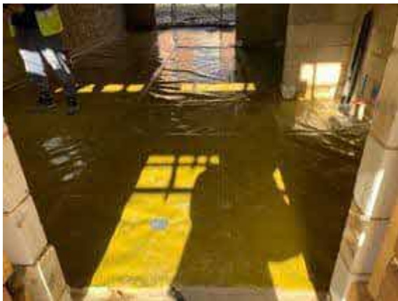
Plot 43 overview of installed membrane.
