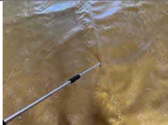
Plot 29 - Air lance integrity test upon a hand welded membrane lap joint.
