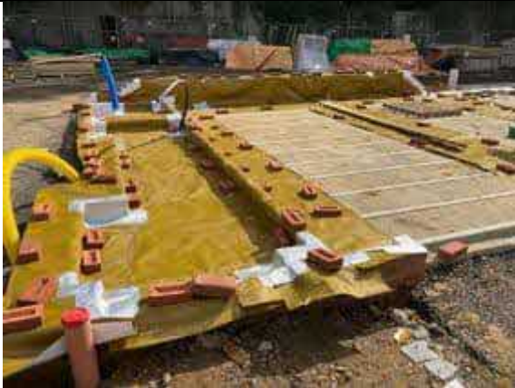
Plot 63 FOG Unit - Overview of Installation of Visqueen Ultimate HC Blok.
