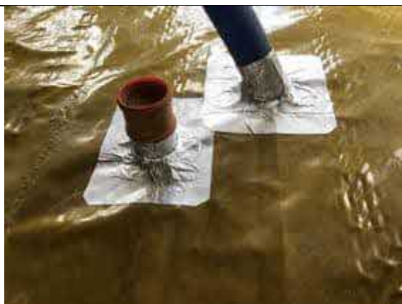
Plot 35 typical double pipe penetration seal using SAGM.
