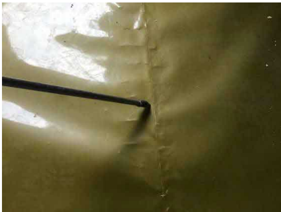
Air lancing all hand welded membrane laps.
