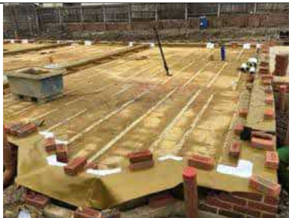
Plot 7 overview of installed membrane.
