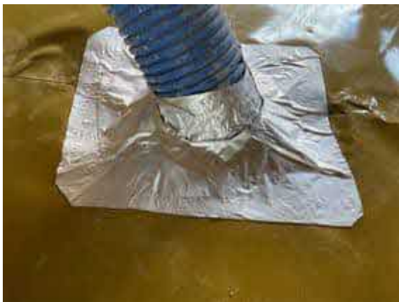
Plot 40. Typical pipe penetration sealed using SAGM.
