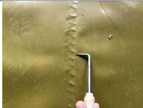
Pick testing all hand welded membrane laps in plot 51.
