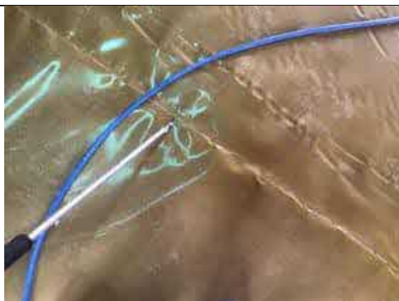
Plot 9 hand welded joint being air lanced
