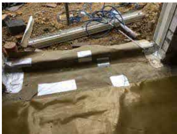
Plot 75 repaired damaged membrane using SAGM.
