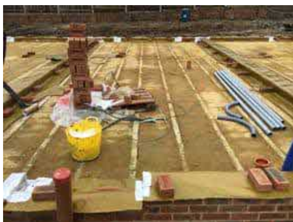
Plot 6 overview of installed membrane.
