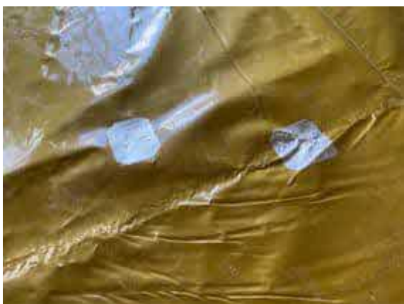
Plot 30 - Patch repairs using SAGM.
