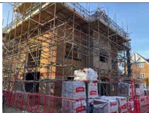
Plot 74 Overview where installation took place.
