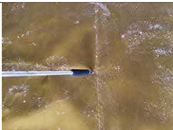
Air lancing all hand welded membrane laps.
