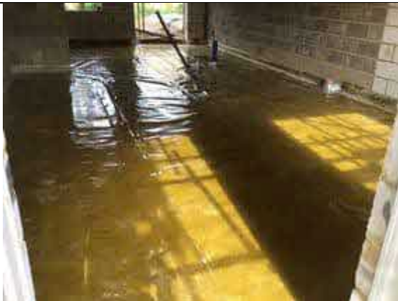
Plot 7 overview of installed membrane.
