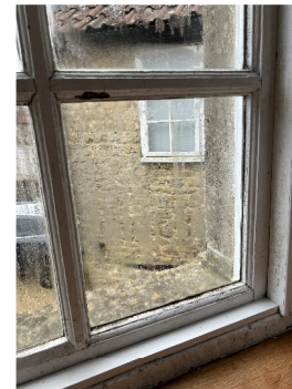
WF.01 bottom rail to lower opening casement two sections of moulded glazing bar have been replaced with square section
