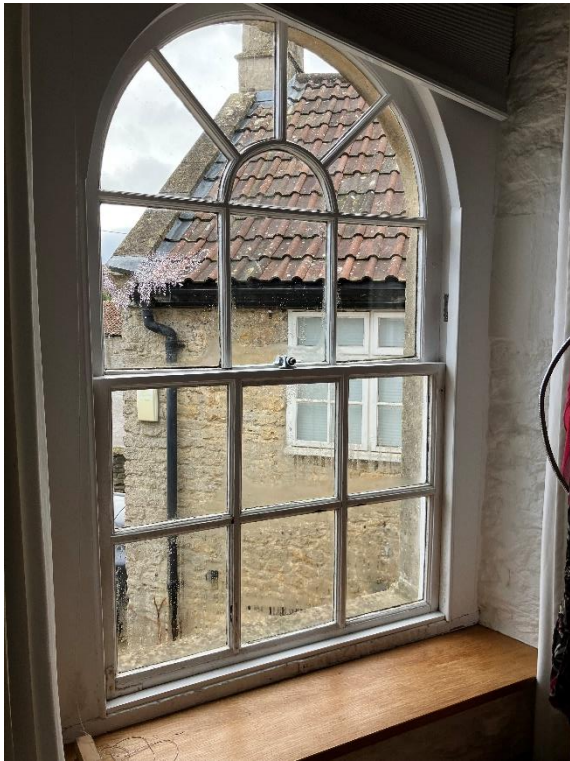
Fig. C.1 First floor courtyard window - interior
