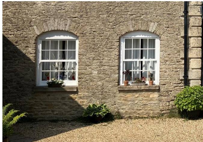
Fig.6 Ground floor courtyard middle and right hand windows
