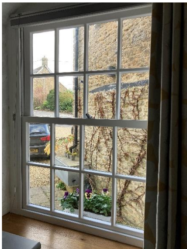
Fig. D.4 Window WG.01 - interior
