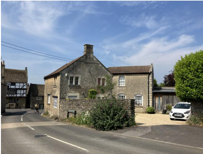
Fig. 3 View looking south-west into courtyard
