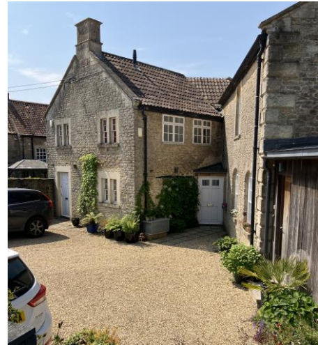
Fig.4 View looking south within courtyard
