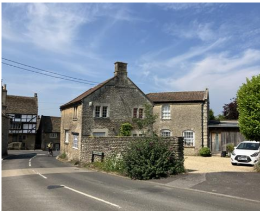
Fig.1 View looking south-west into courtyard
