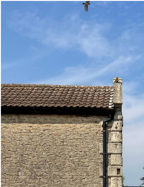
Fig.3 Mortar bedding to ridge tiles and lead flashing to verge parapet
