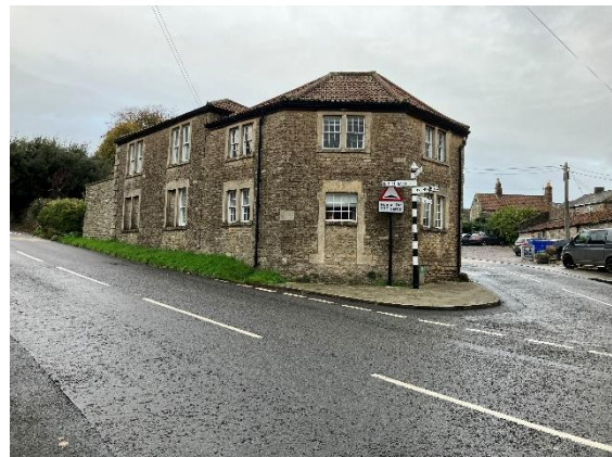
Fig.2 View looking north-east toward Farleigh Road
