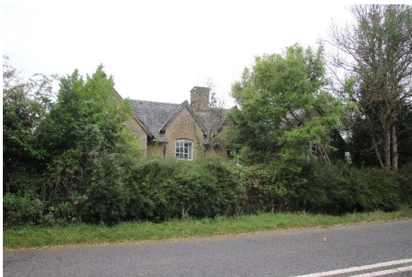
3. House from the north-east
