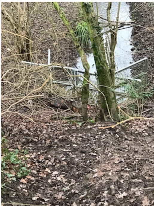
Debris protection measures at river behind property
