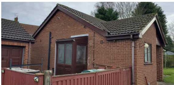
3 Side – north west aspect
