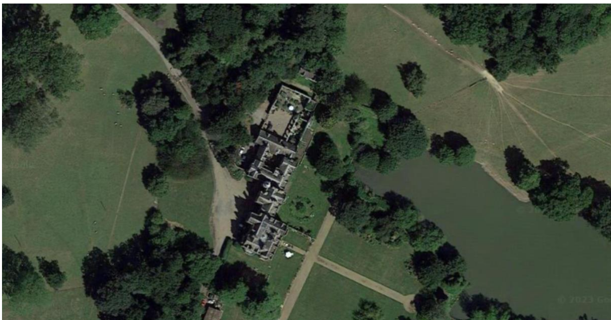
Figure 2, Aerial view of Rauceby Hall.
