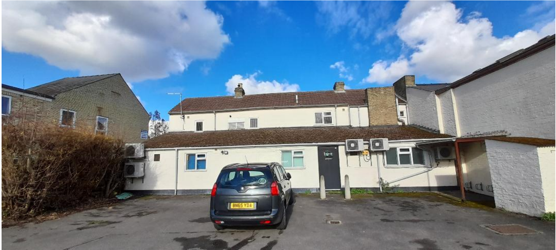
View from rear carpark.
