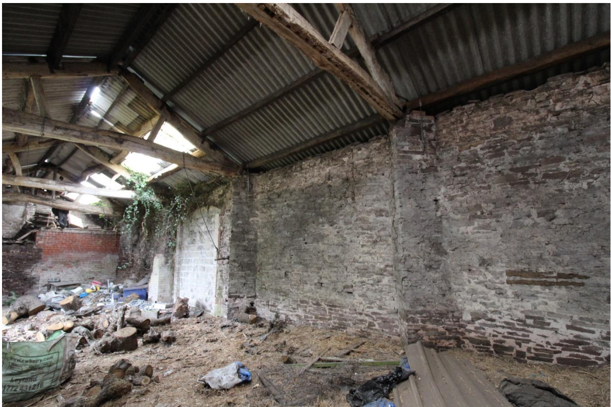
Plate 47 – Main Barn Range East Wall
