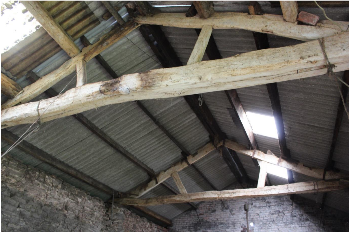
Plate 44 – Main Barn Range (Looking South)
