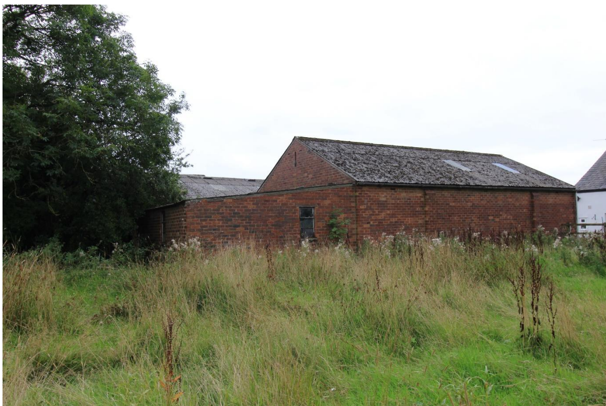
Plate 53 – Outbuilding to North of Farmhouse
