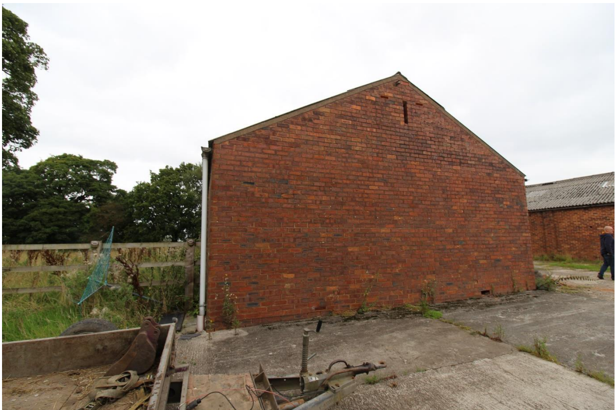
Plate 55 – Outbuilding to North of Farmhouse
