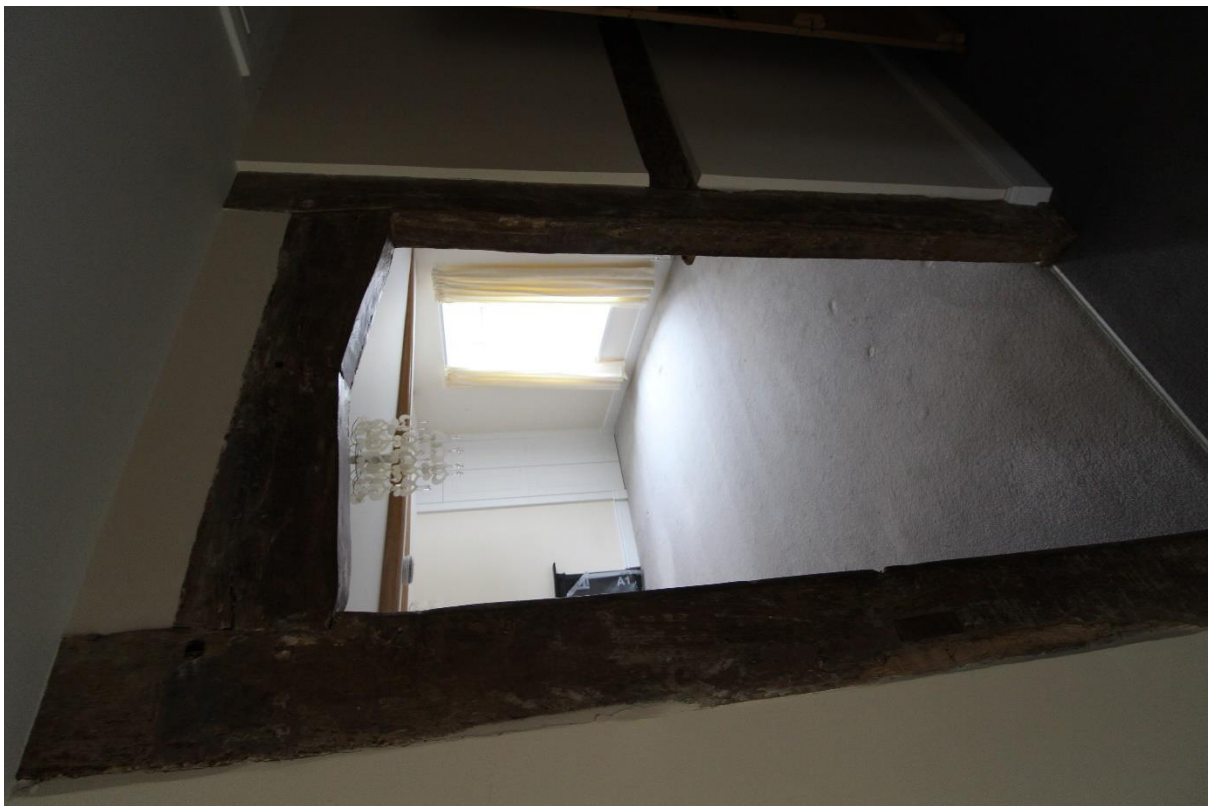
Plate 21 – Room 8 (Looking into Room 11)
