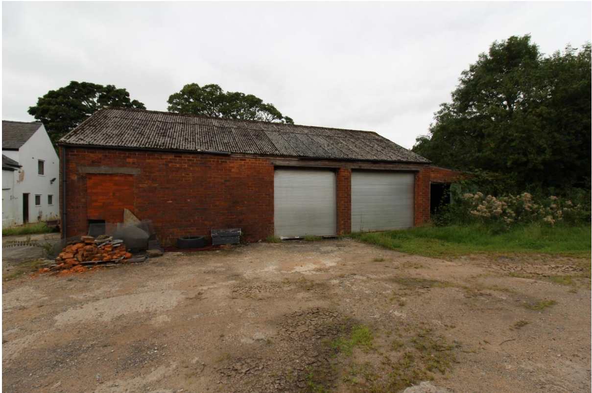
Plate 54 – Outbuilding to North of Farmhouse
