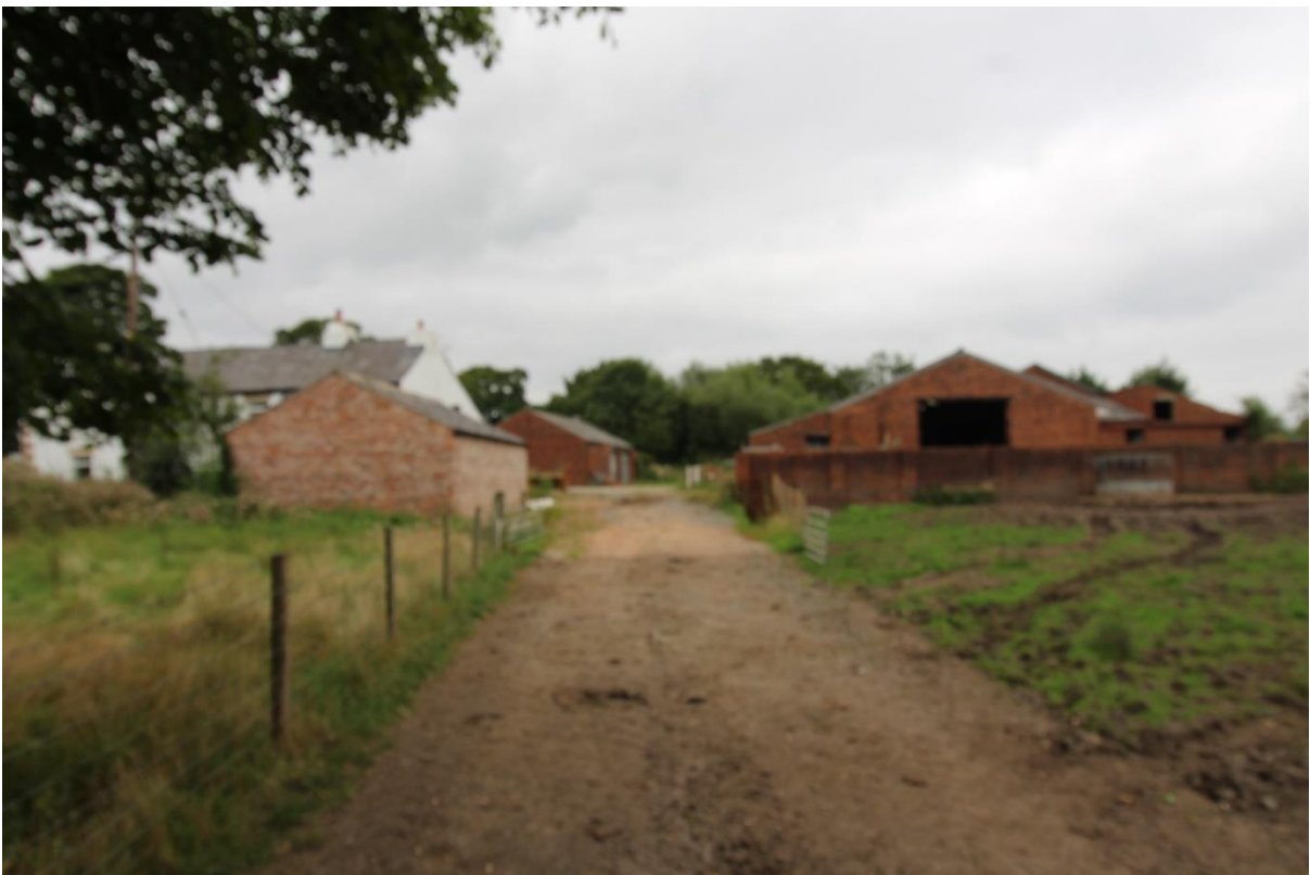
Plate 57 – Complex From Access Road
