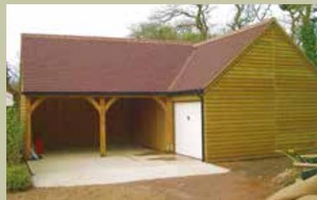
L shaped 2 Bay Carriage House, Workshop and Garage
