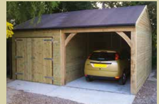
1 bay Carriage House with attached Garage. 22° felt roof.
