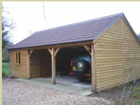
2 bay Carriage House with attached Workshop. 30° interlocking concrete tile roof.
