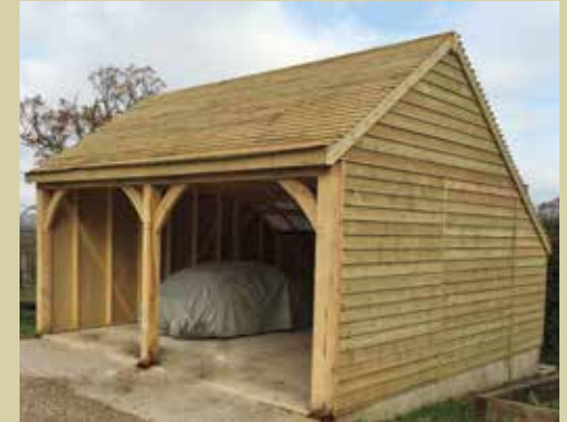
5.4 x 5.4 two bay Open Barn. 35° Battened and felted, awaiting tiles.
