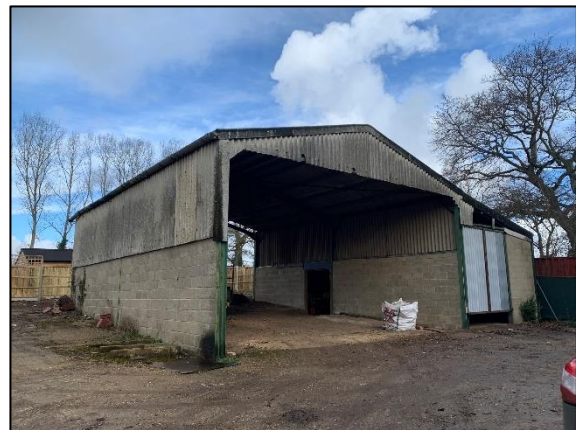
Figure 2. Looking north-west across site
