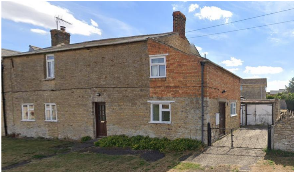
Figure 1 House as Existing
