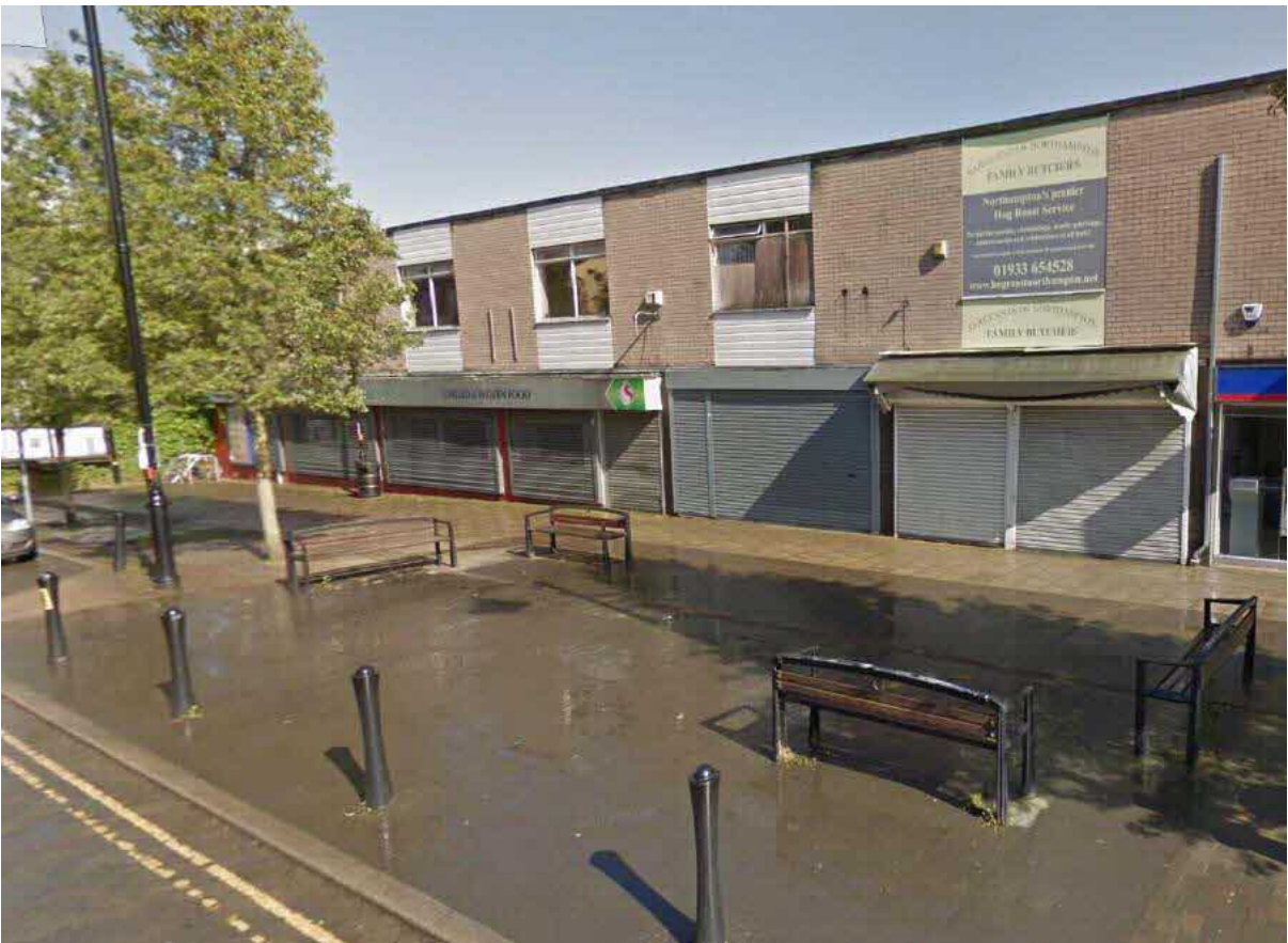
View from High Street
