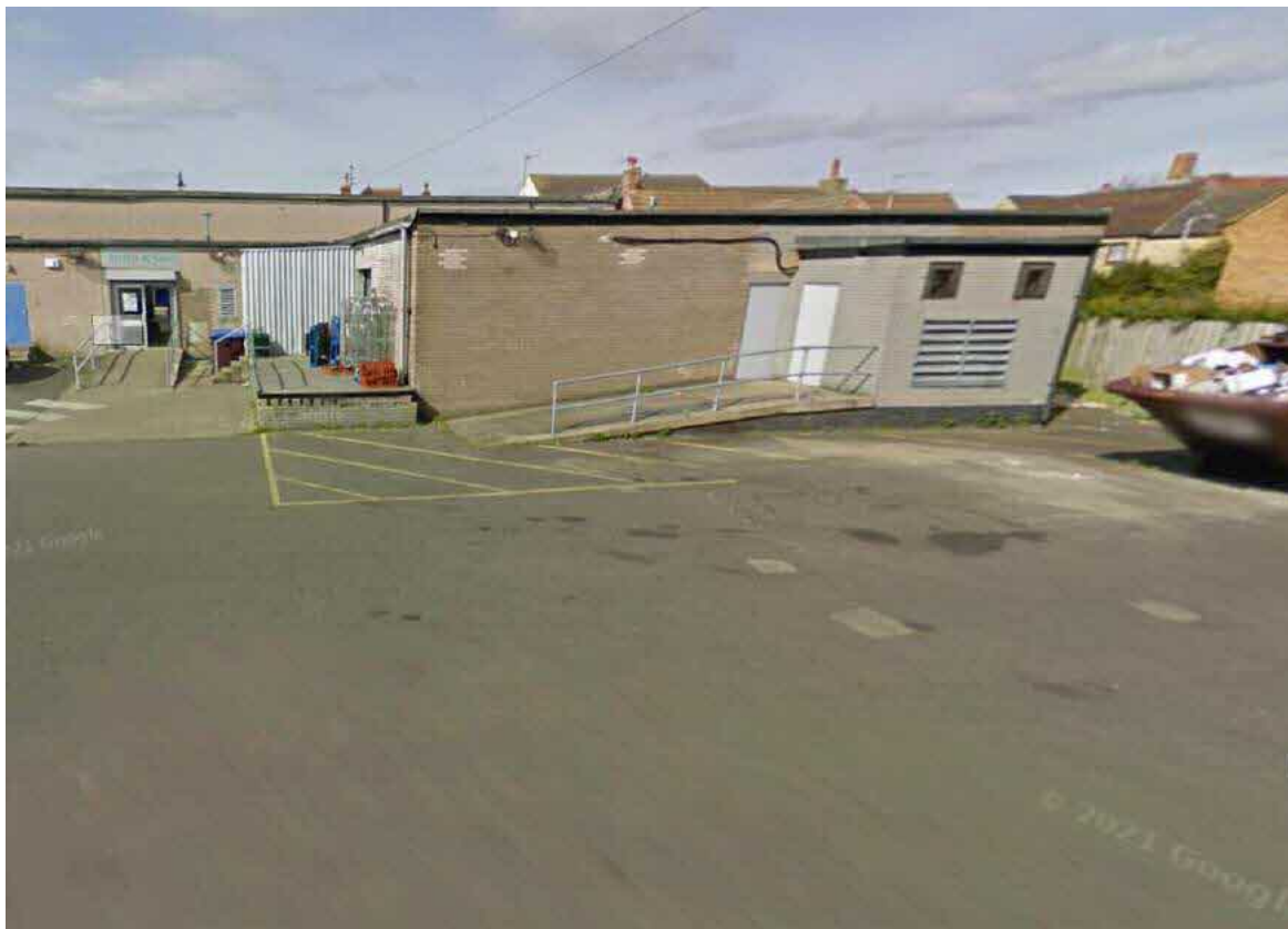
View to rear of 13-21 High Street
