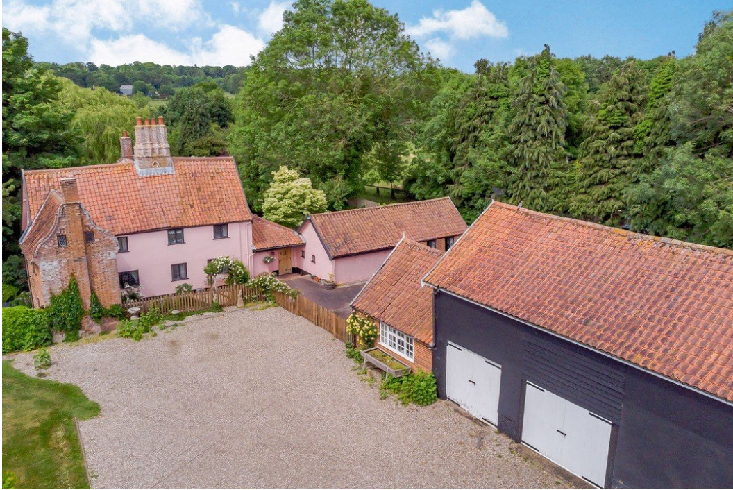
Photograph 1 - existing asphalt visible to right of picture, picket fence visible to front of house all now removed.
