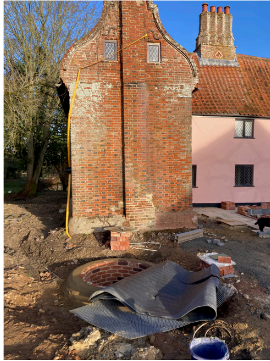
Photograph 3 - well in context to south facing gable
