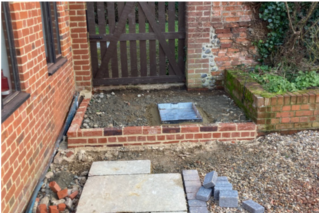
Photograph 6 - replacement step, set away from house to reduce damp ingress.
