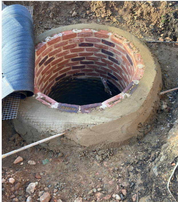
Photograph 2 - discovered well, raised to ground level, it is proposed to raise this around 600mm above ground.
