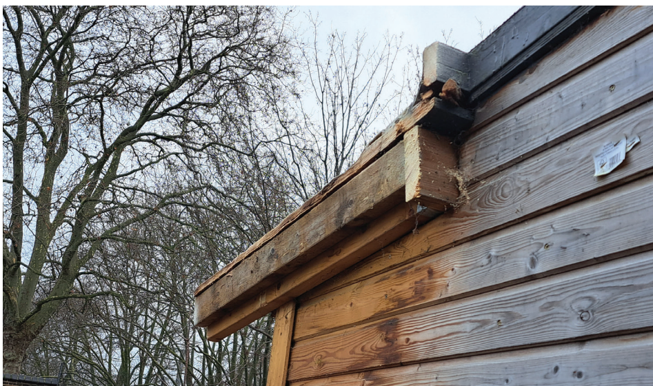
Rear extension : CANOPY REMOVED (December 2023)
