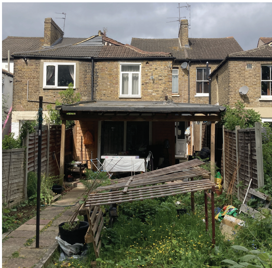
Rear extension and its canopy (June 2023)
