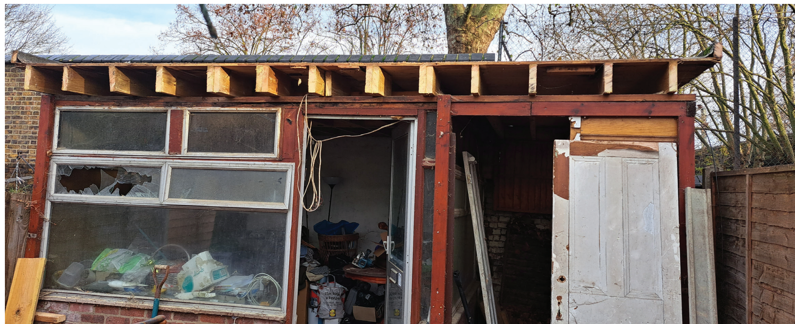
Canopy to outbuilding : REMOVED (December2023)
