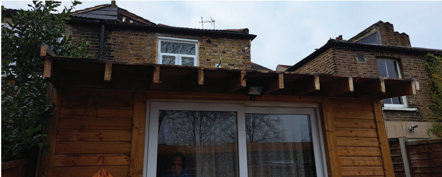
Rear extension : CANOPY REMOVED (December 2023)
