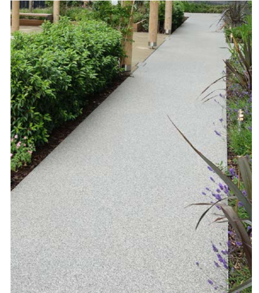
Metal edging to the resin bound gravel paving
