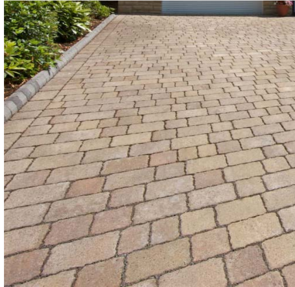
Permeable block paving to turning area
