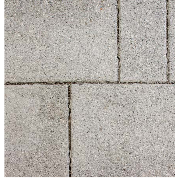
Permeable flag paving to entrances
