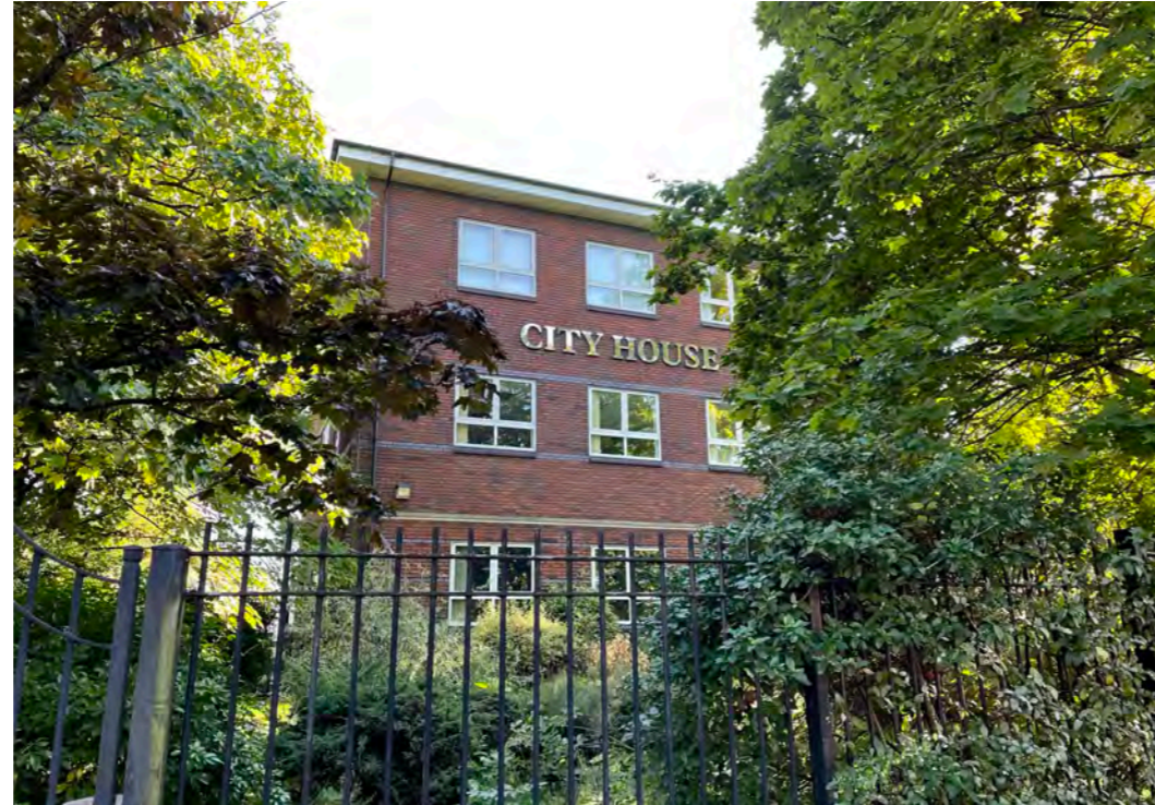
Figure 1.2 City House, taken on Site visit from pavement of Cheam Road
