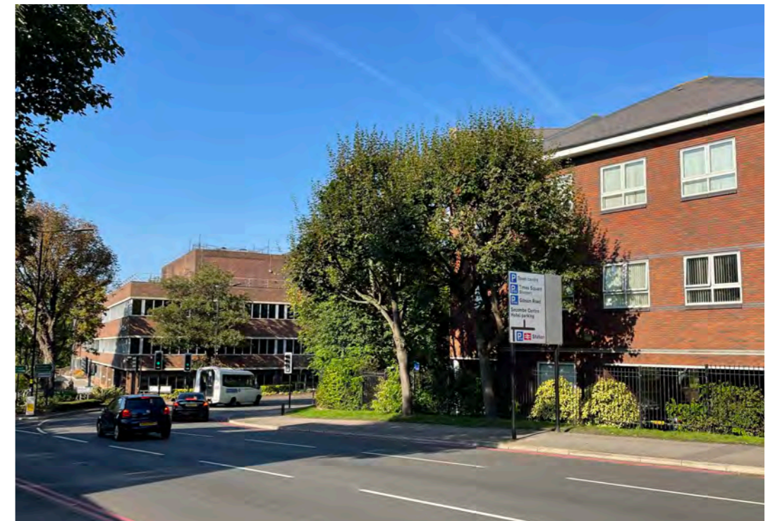
Figure 1.5 The side flank of City House, taken on Site visit
