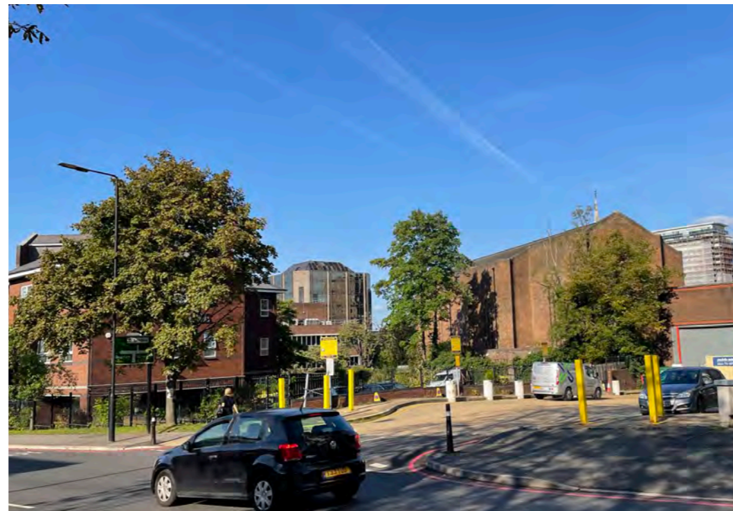
Figure 1.4 The rear of City House, taken on Site visit. Baptist Church seen in the right of the frame.
