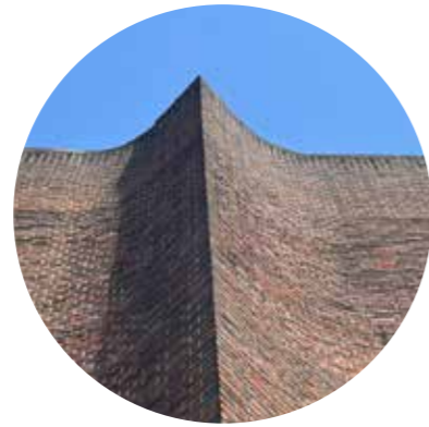
Curved Brick Piers
