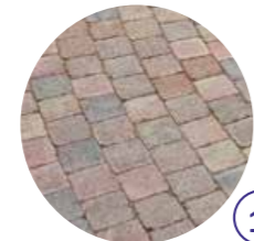
1 Permeable block paving for vehicular access
