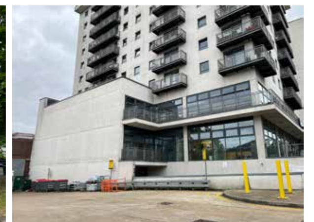
Neighbouring Building Mixed-use building to the south 2-6 Sutton Park Road
