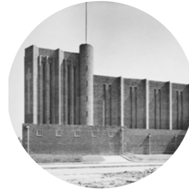
Piers accentuating verticality
