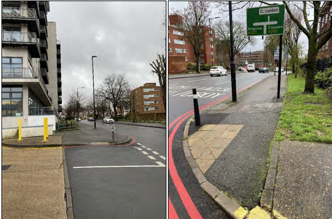
Photograph's 3 and 4 Footway Provision
