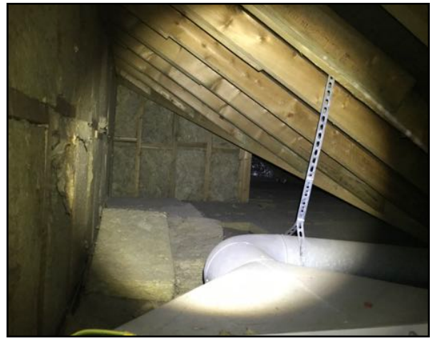
Image 13: View of loft void two.
