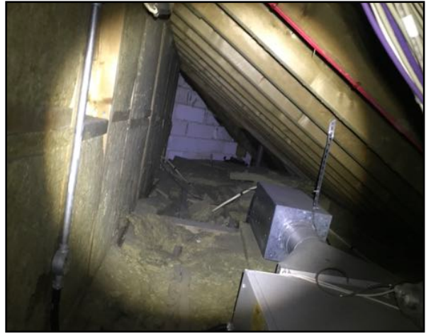
Image 11: Internal view of loft void one.
