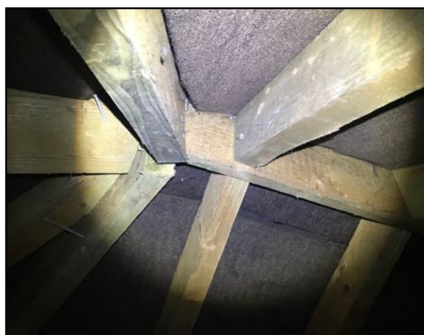
Image 15: Central ridge beam in loft void three.
