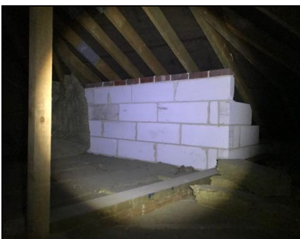
Image 14: View of loft void three.
