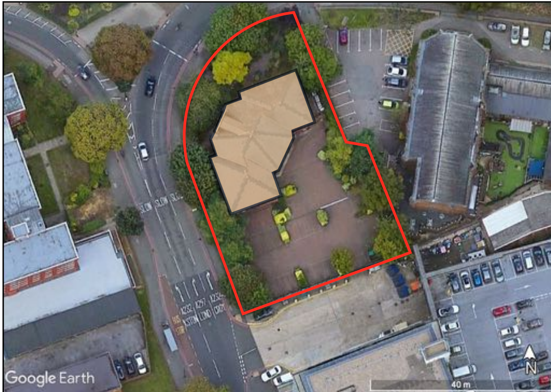
Figure 1: Site location within the local landscape (Copyright Google Earth Pro, 2023). The building subject to survey is highlighted in orange.
