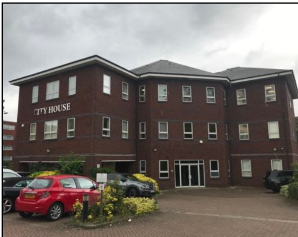
Image 6: View of the southern elevations of the building.
