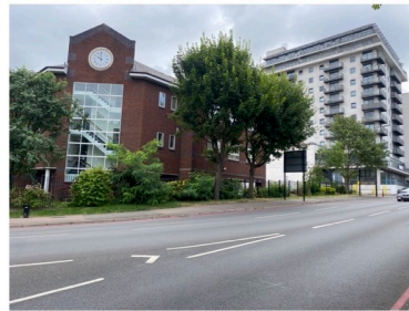
Front of site / western boundary trees T7-T11 viewed to south
