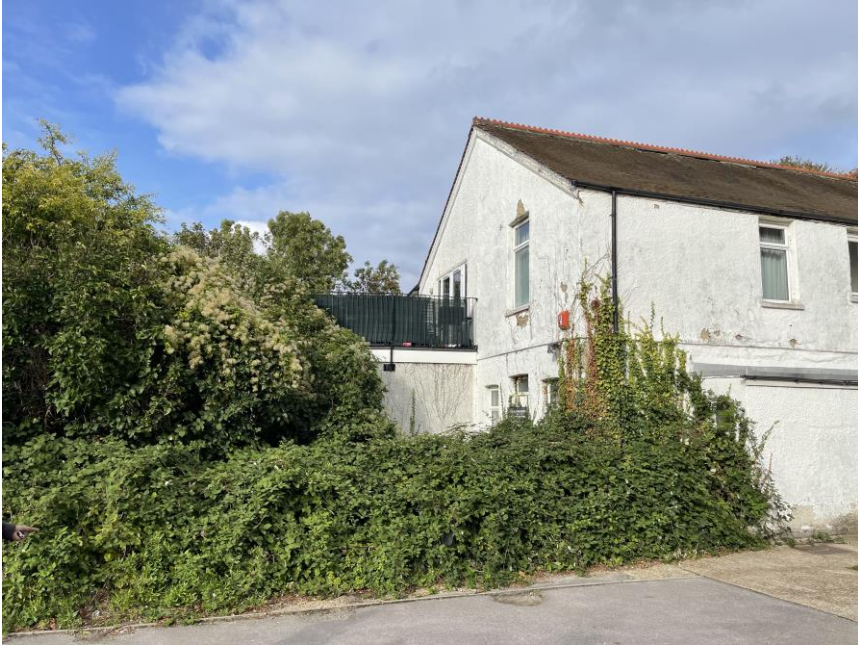
Figure 3: Side Views of the building with no. 5 rear single storey and rear terrace.
