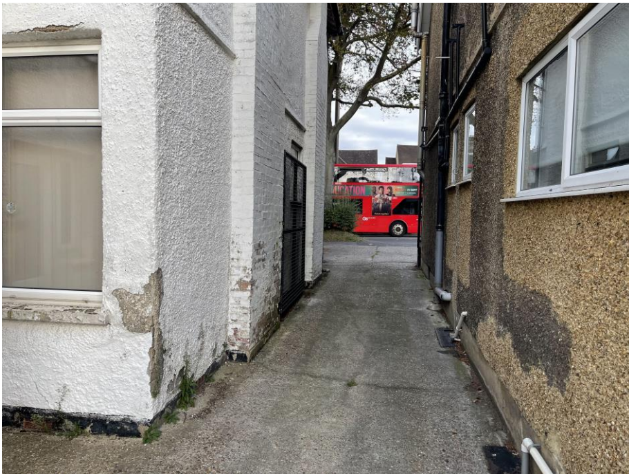
Figure 3: View of shared drive between no. 7 & 9 Beeches Avenue.
