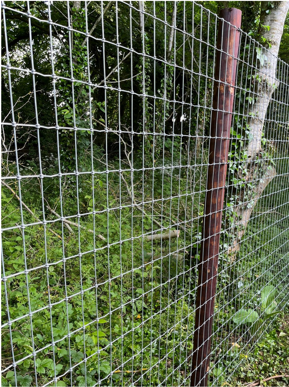
Example of the proposed 1800 high post and wire mesh fence to be installed
