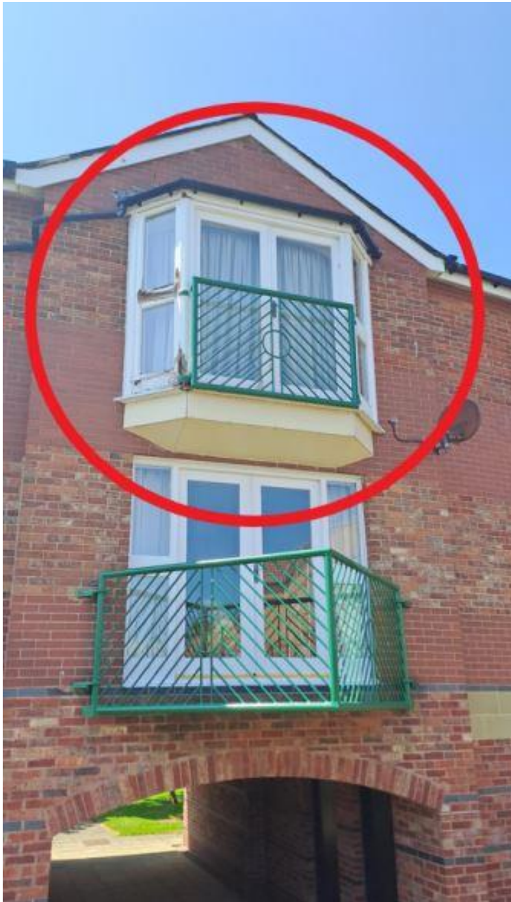
3. 3 Ensign House, central bay window and doors, east elevation, second floor (3)
