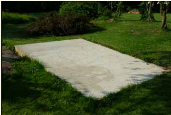
Example concrete base for a cedar greenhouse
