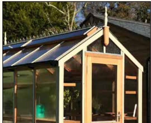
Aluminium cladding on gable rafters and corner posts
