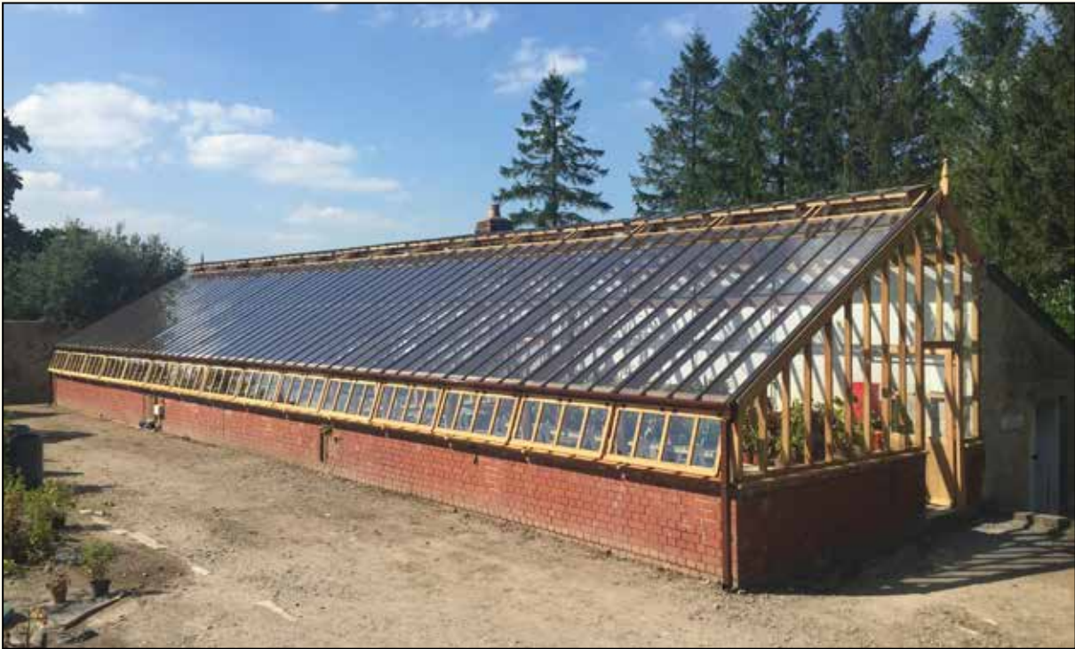
Delivered and installed in North Somerset. Size: 17ft x 75ft
