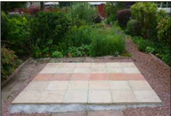
Example slabbed base for a cedar greenhouse
