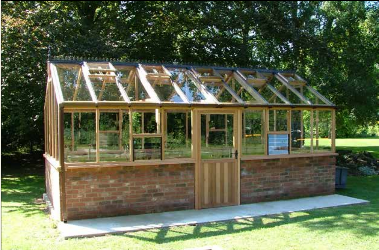
Delivered and installed in Cambridgeshire. Colour—Clear. Size: 10ft x 20ft
