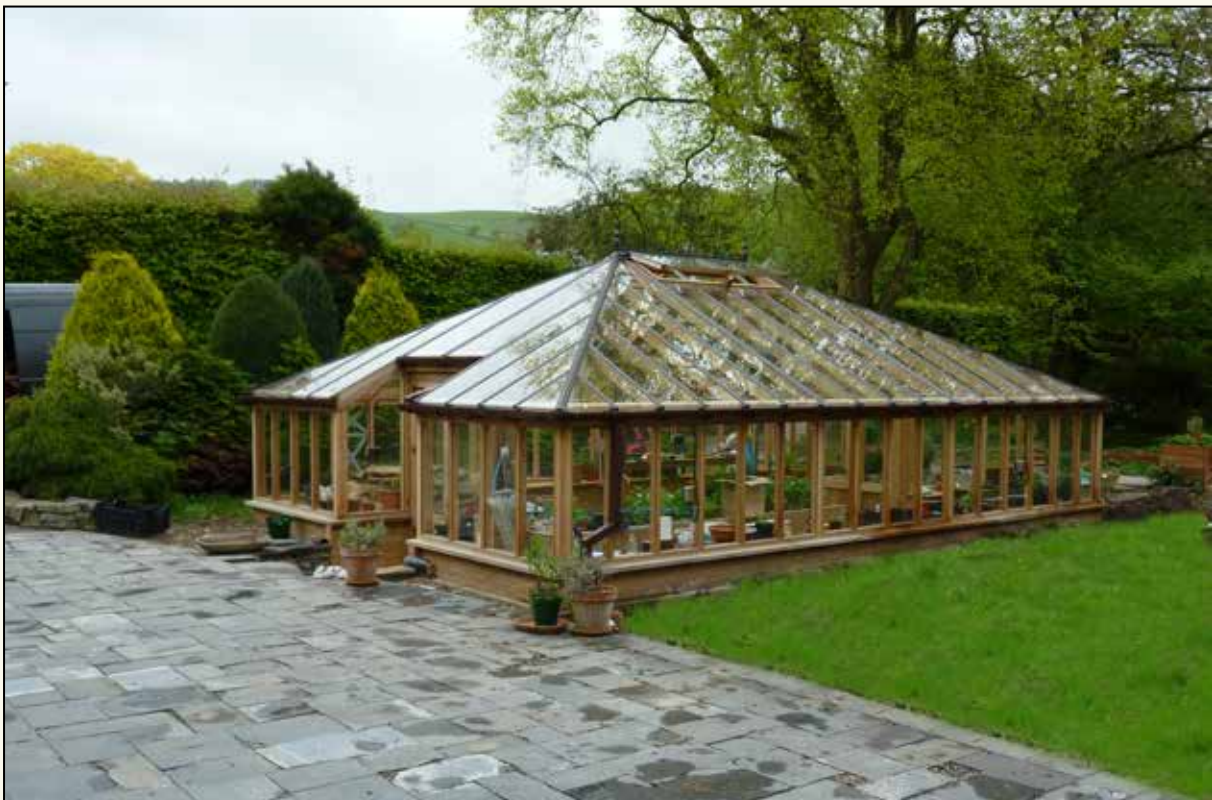
Delivered and installed in Lancashire Colour—Clear. Size: 18ft x 28ft
