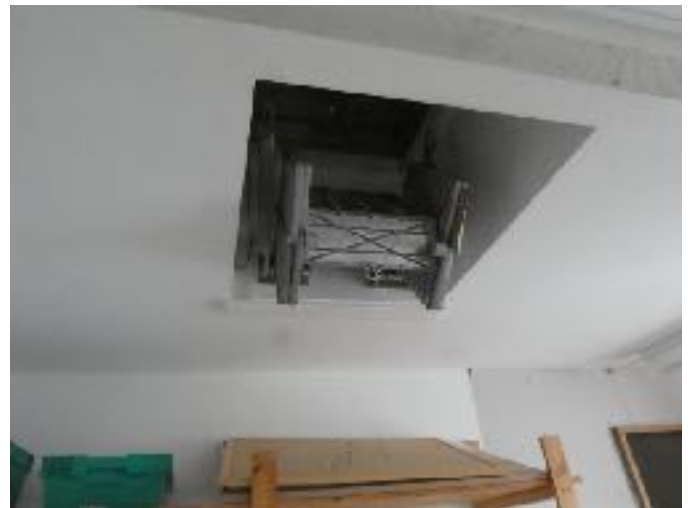
Existing room 22 no works undertaken yet
