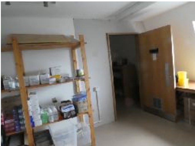
Existing room 21 no works undertaken yet
