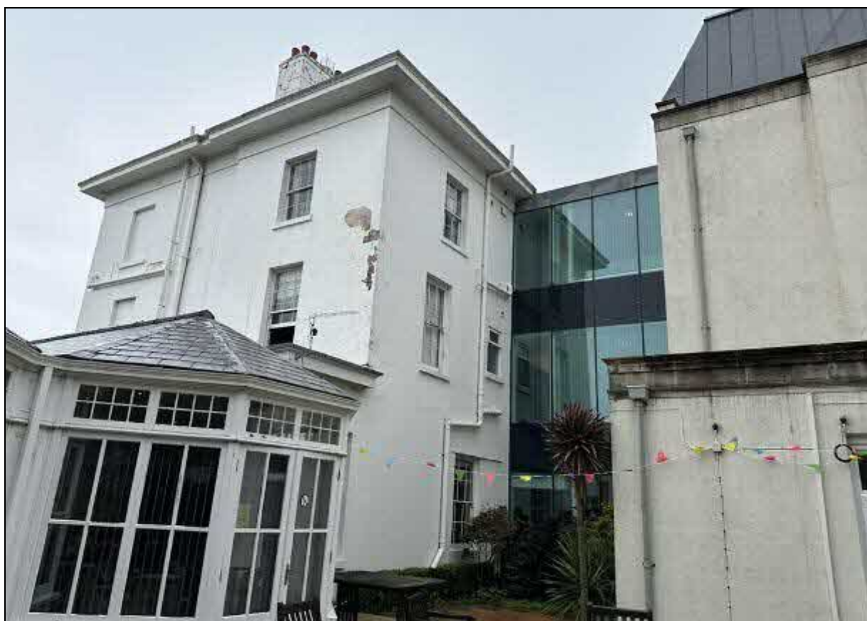
6. A glass link separates the original building from the wing: view from within the site
