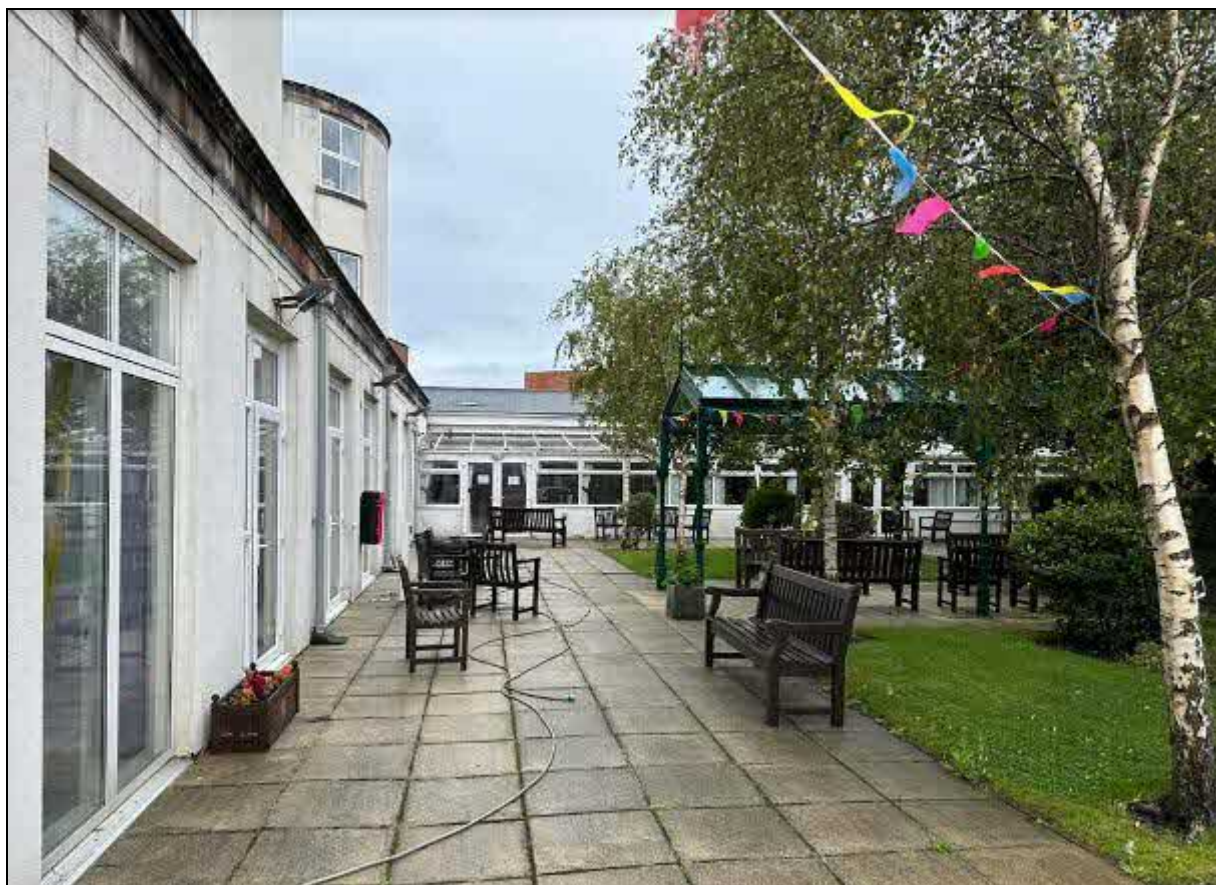
7. The single storey Frankenburger wing, at right angles to the 2007 wing
