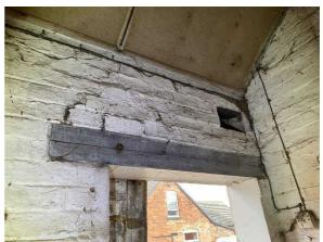
Internally, a combination of brick and blockwork walls divide the space. Partition walls are largely in acceptable condition with no signs of significant structural stress to raise concern. The exception being partition walls directly adjacent to those areas affected by roof spread. Localised rebuilding of partition walls, where they abut external walls, is required to address cracking.
