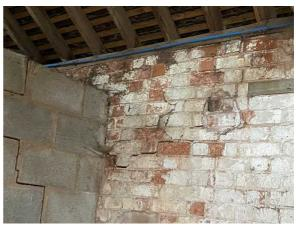
Localised areas of recessed pointing were identified throughout the building, which would benefit from re-pointing in a lime-based mortar. Additionally, spalling of brickwork was also noted in small areas. Isolated replacement of the most severely affected bricks would be considered beneficial.
