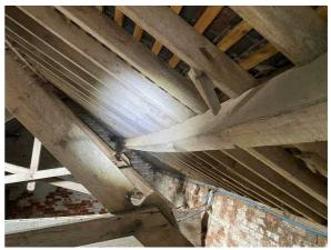
Water ingress via the centre roof light has resulted in visible staining of the adjacent purlin and is likely to have caused a degree of timber decay. At the til inspection the structural integrity of the purlin did not appear to have significantly compromised; however, localised minor repair works should be anticipated.
