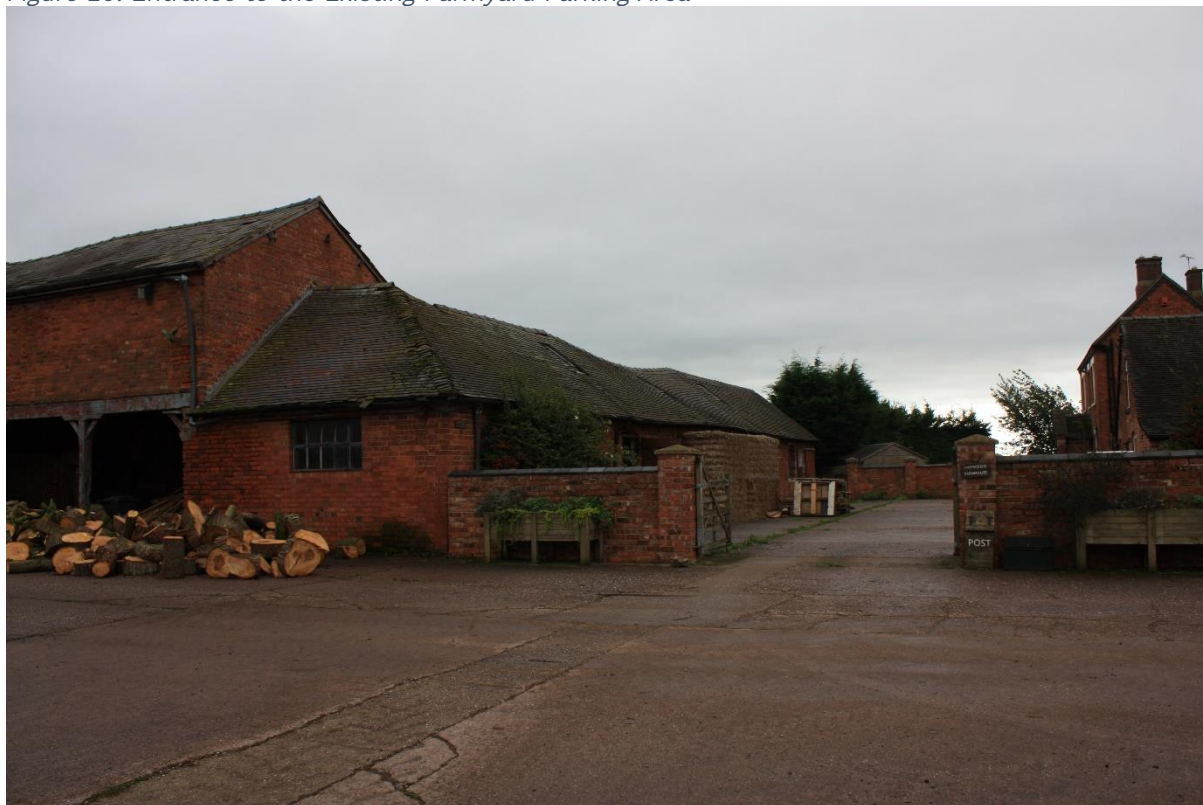
Figure 20: Entrance to the Existing Farmyard Parking Area
