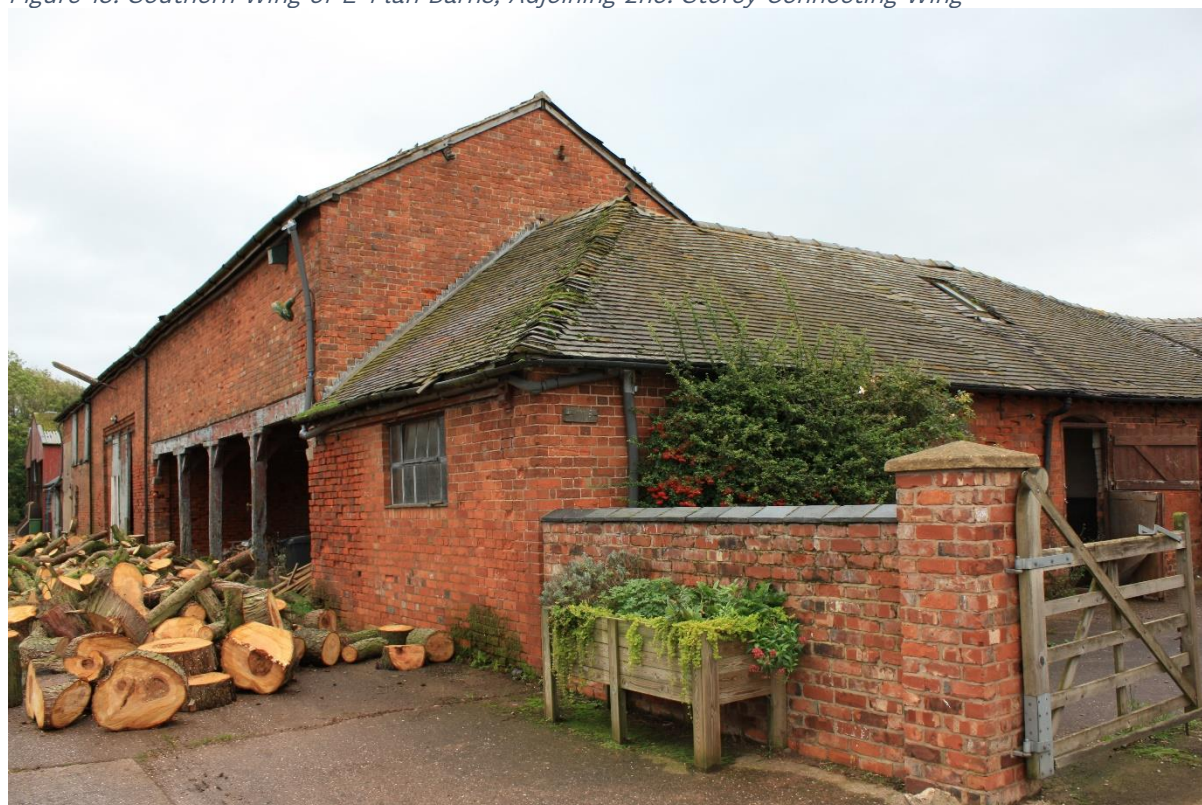
Figure 13: Southern Wing of E-Plan Barns, Adjoining 2no. Storey Connecting Wing
