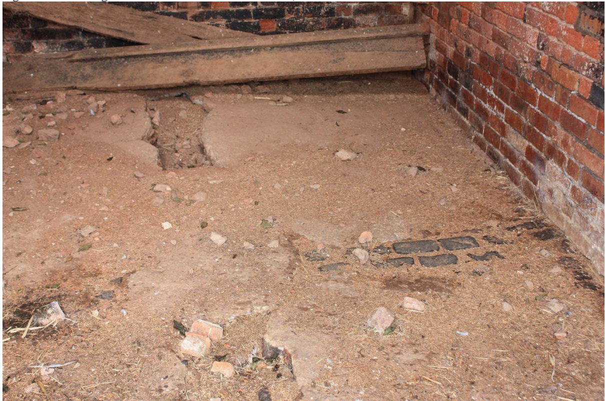
Figure 18: Existing Concrete Slab over Brick Floor, Part of Which Has Since Been Removed.
