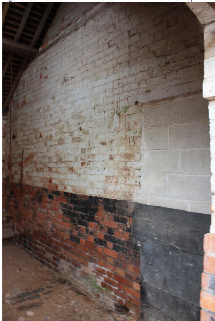
Figure 16: Internal Brick Built Partition with Blocked Up Doorway Proposed for Reopening
