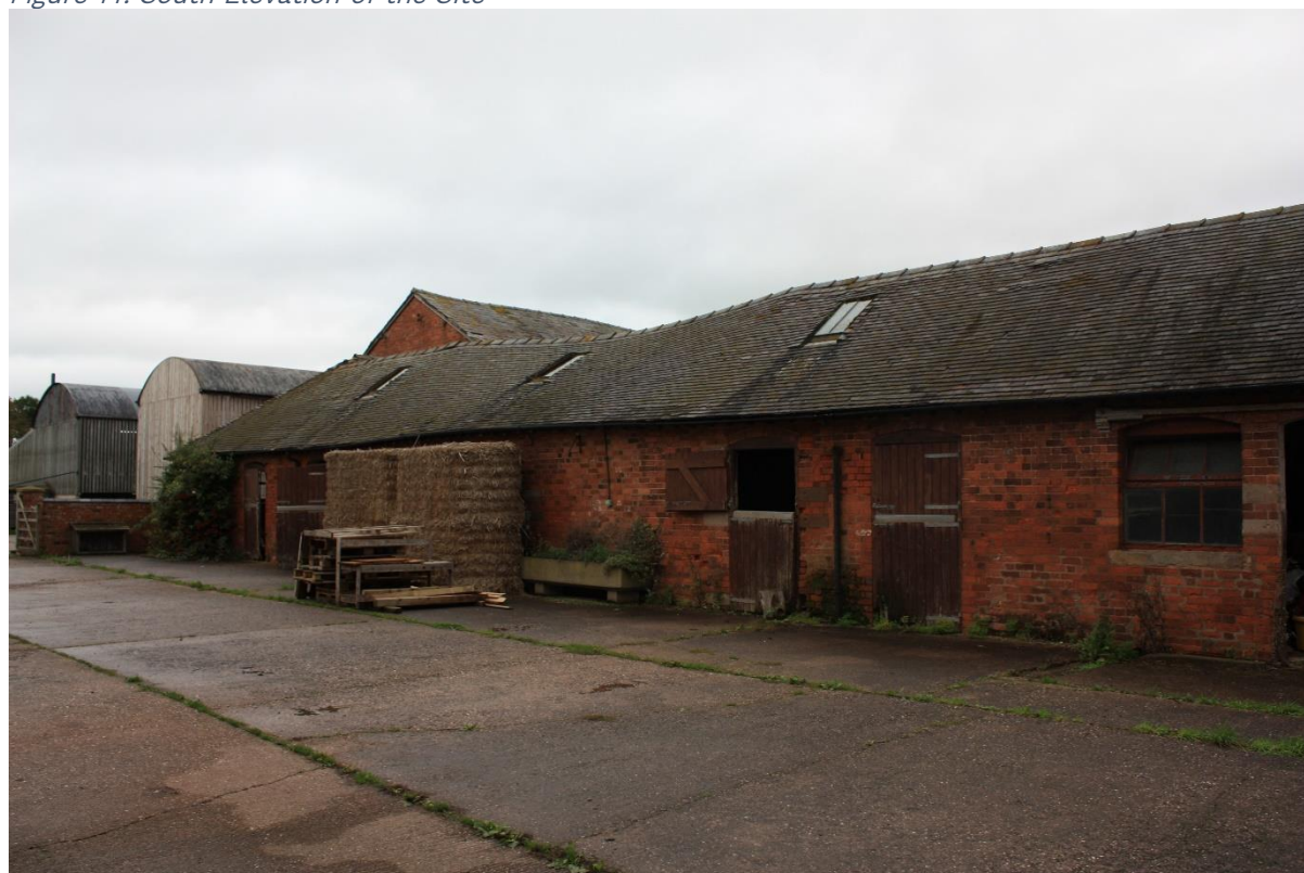
Figure 14: South Elevation of the Site
