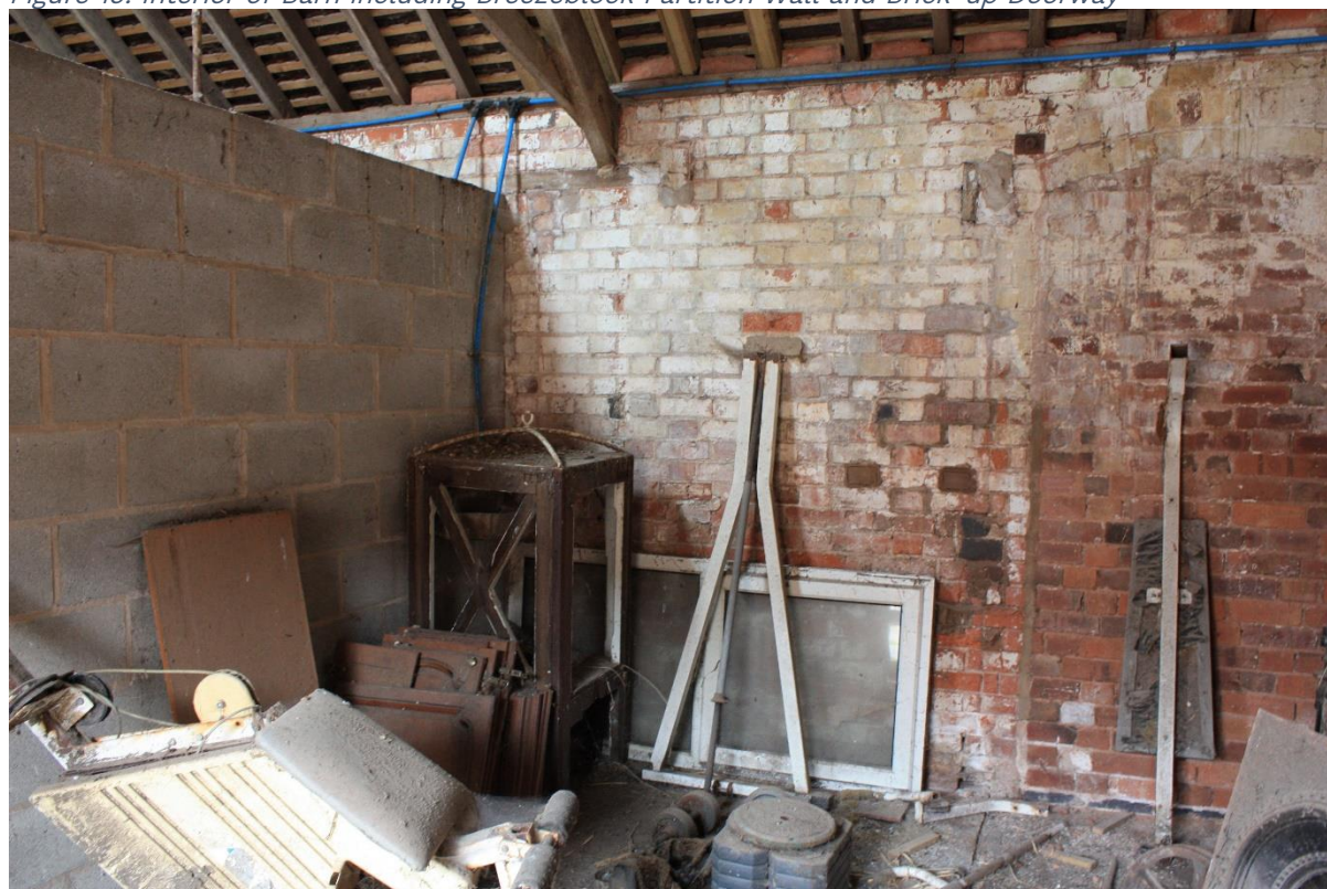
Figure 15: Interior of Barn Including Breezeblock Partition Wall and Brick-up Doorway
