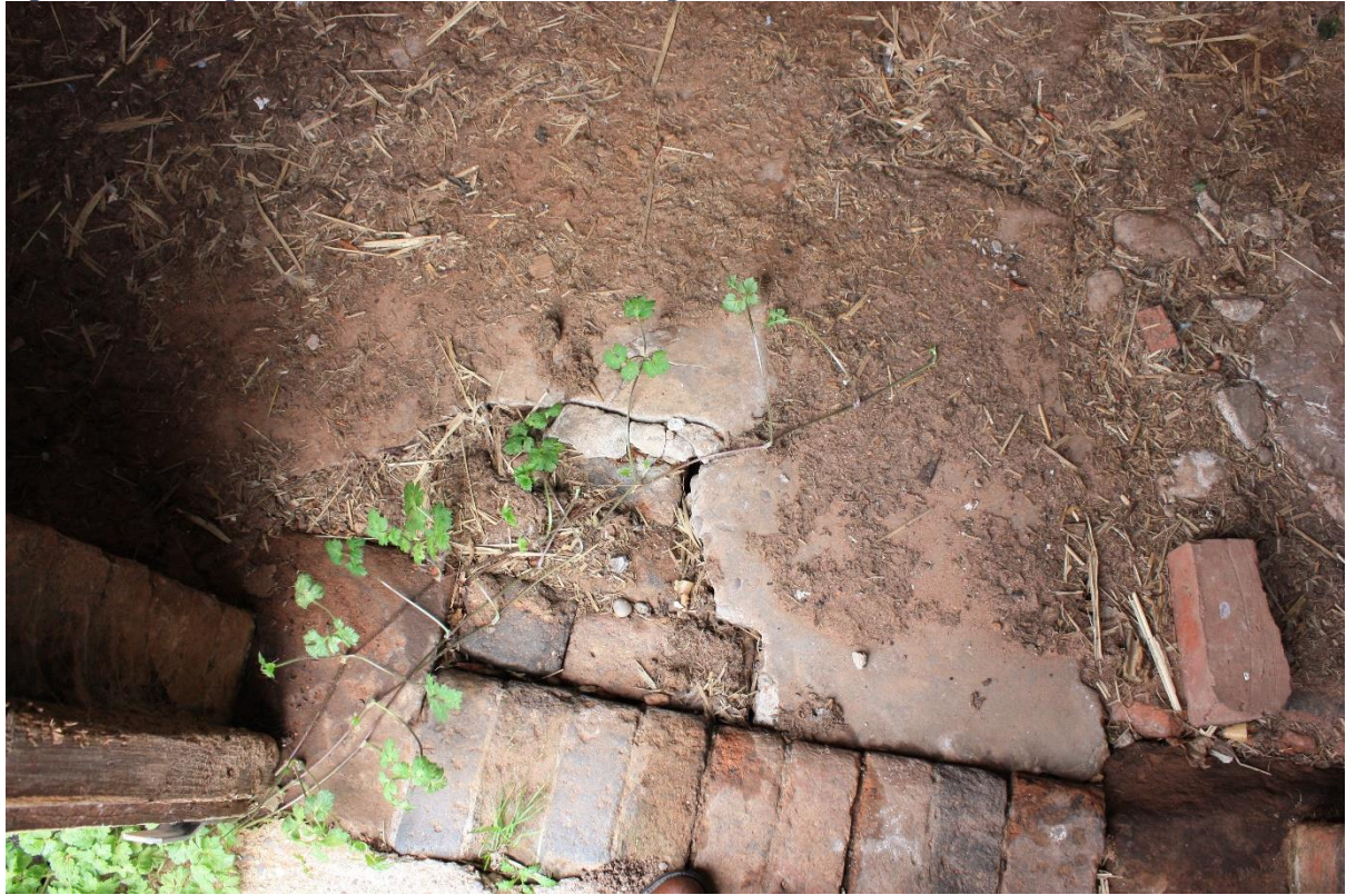
Figure 18: Existing Concrete Slab over Brick Floor, Part of Which Has Since Been Removed.
