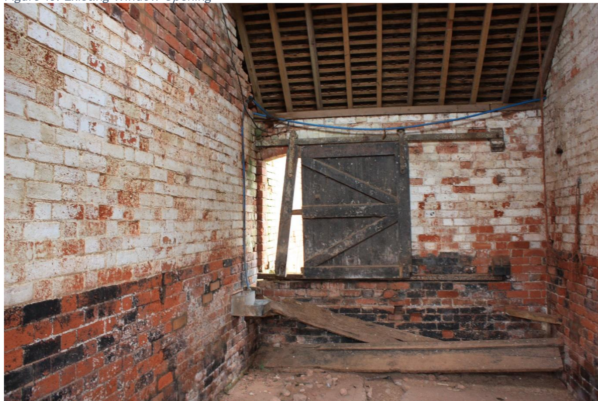
Figure 19: Existing Window Opening
