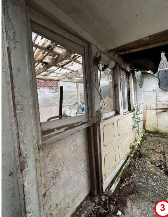
Inside view of the existing annex
