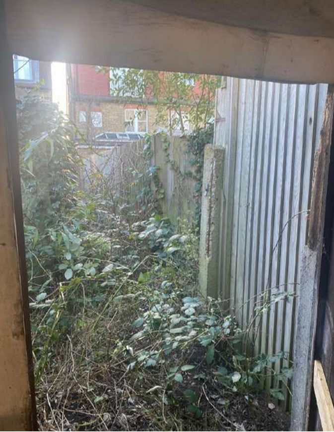
Annex door to rear alleyway
