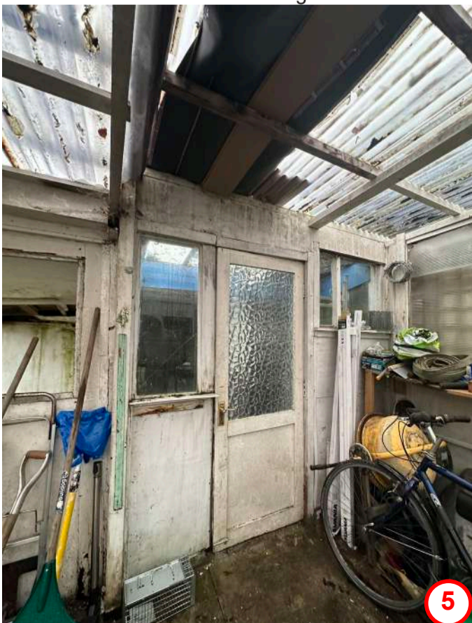
Inside view of the existing annex
