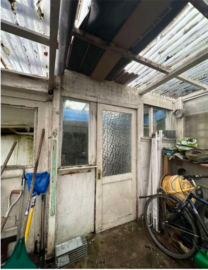
Inside view of the existing annex
