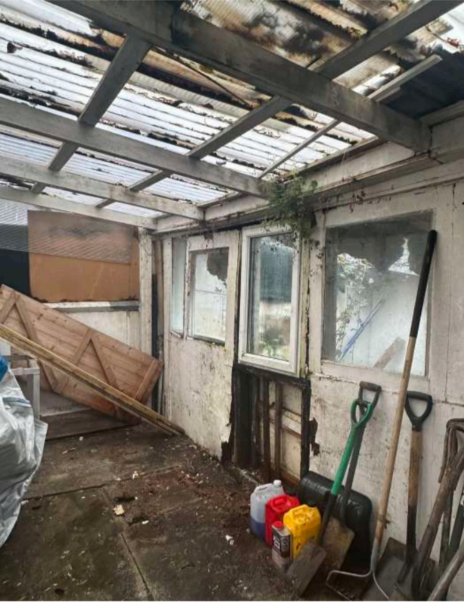
Inside view of the existing annex
