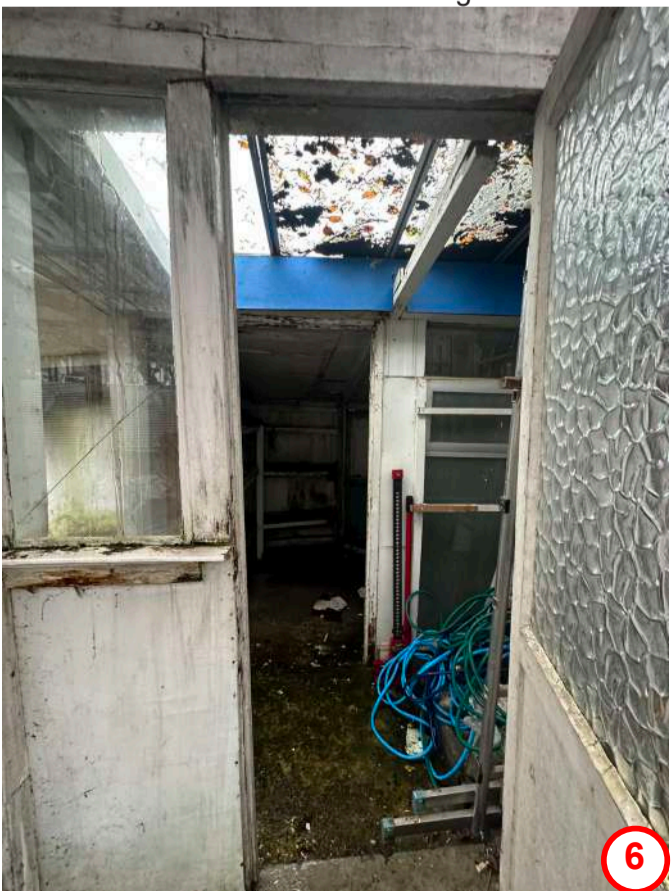
Inside view of the existing annex
