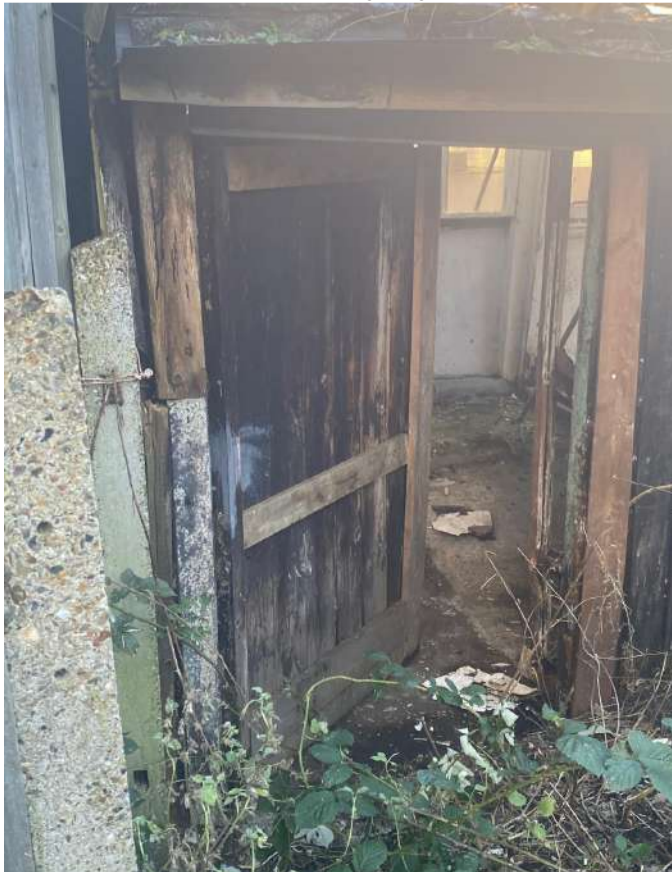
Rear door view from the alleyway
