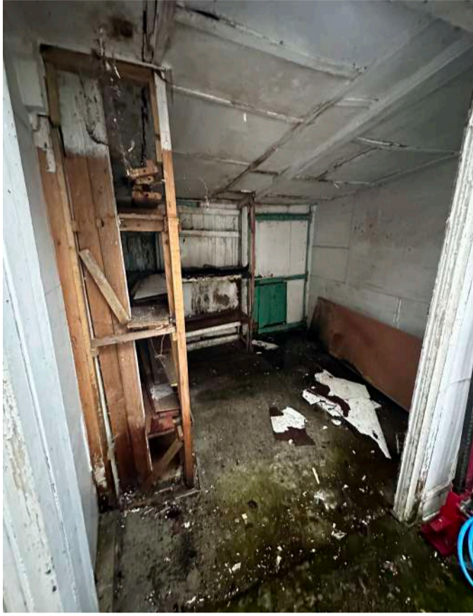
Inside view of the existing annex
