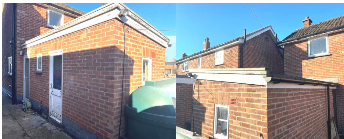
Figure 1- East and south elevations (left), north elevation (right)
