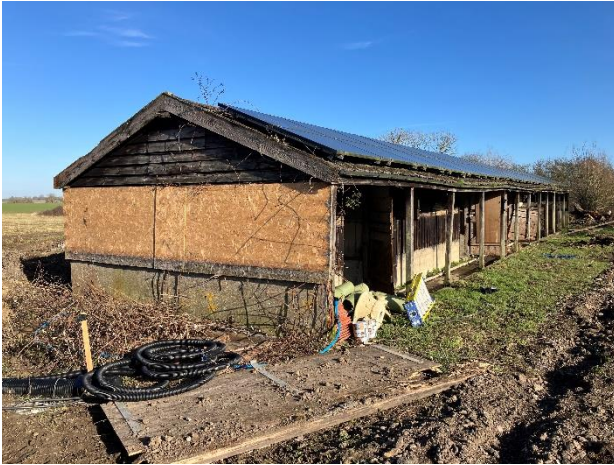
Photo 1: South western facades of building
