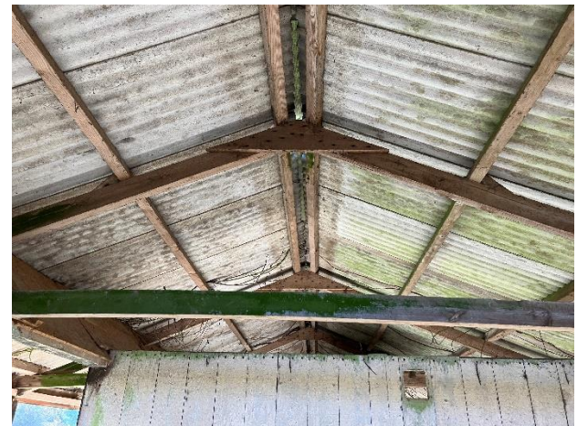
Photo 6: Internal roof structure, with no central ridge beam
