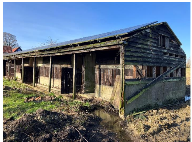
Photo 4: South western facades of building
