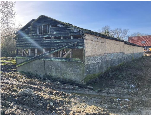
Photo 3: North eastern facades of building
