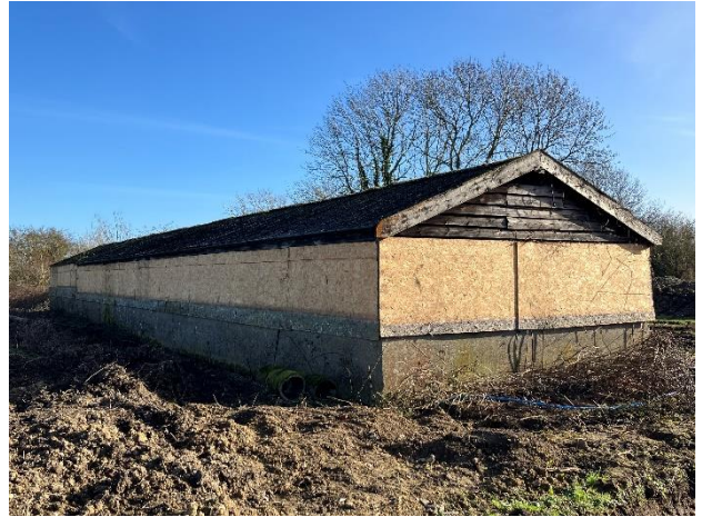
Photo 2: North western facades of building
