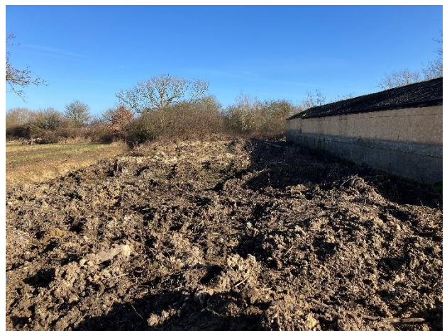
Photo 12: Bare earth to rear (north) of building
