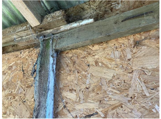
Photo 8: Northern chipboard wall fitting closely to modern wooden frame
