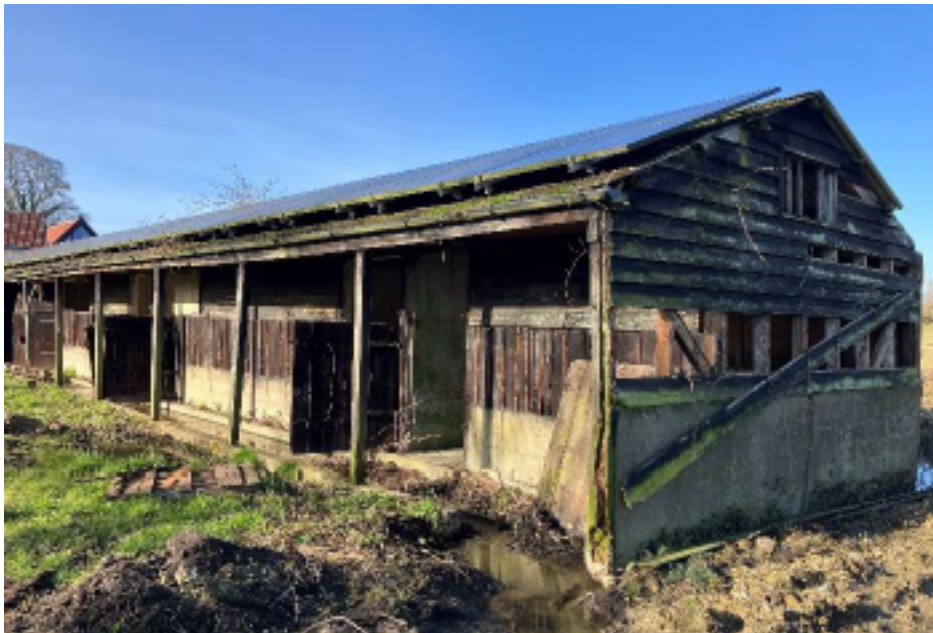
Picture 6 – South western facades of the building
