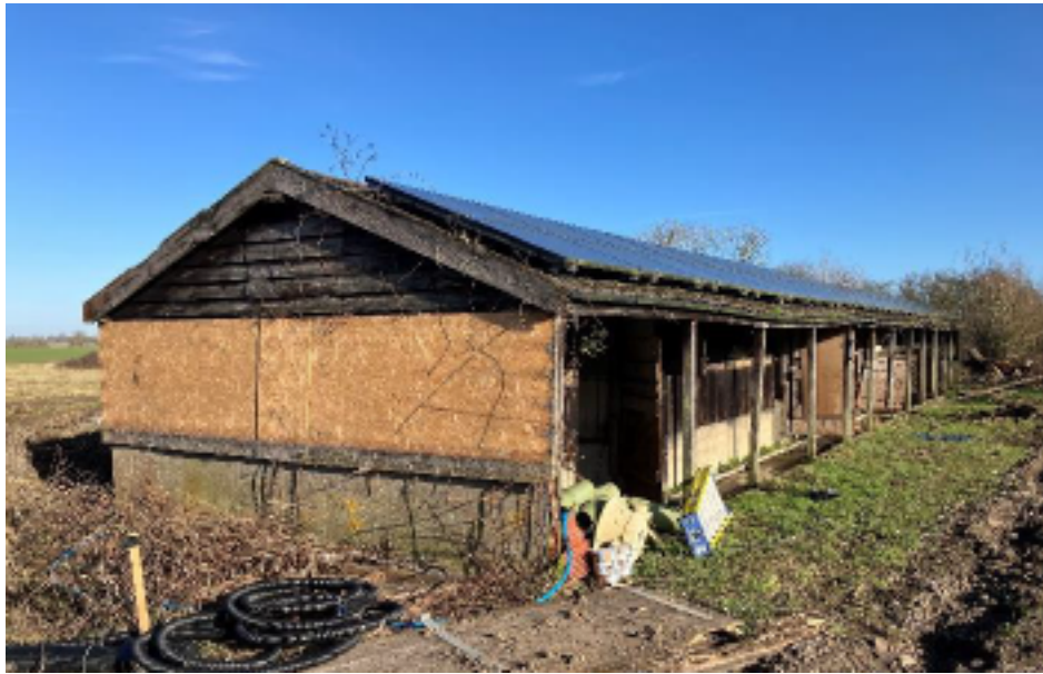
Picture 3 – South western facades of the building
