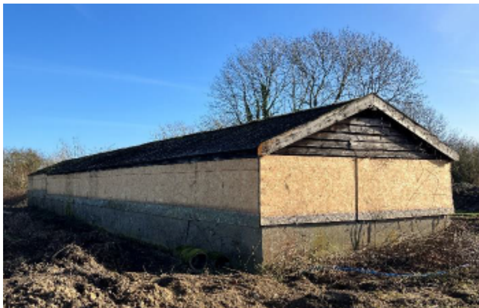
Picture 4 – North western facades of the building
