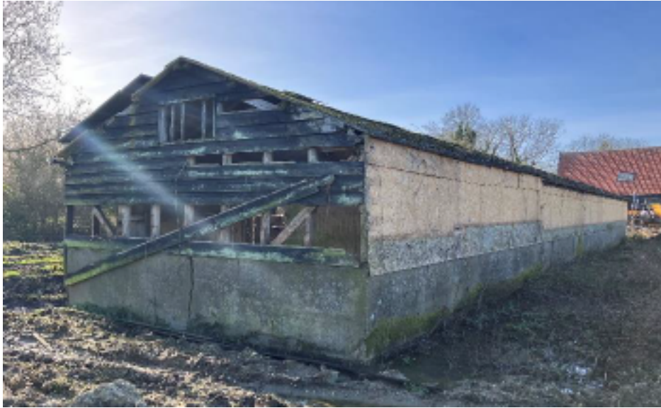
Picture 5 – North eastern facades of the building
