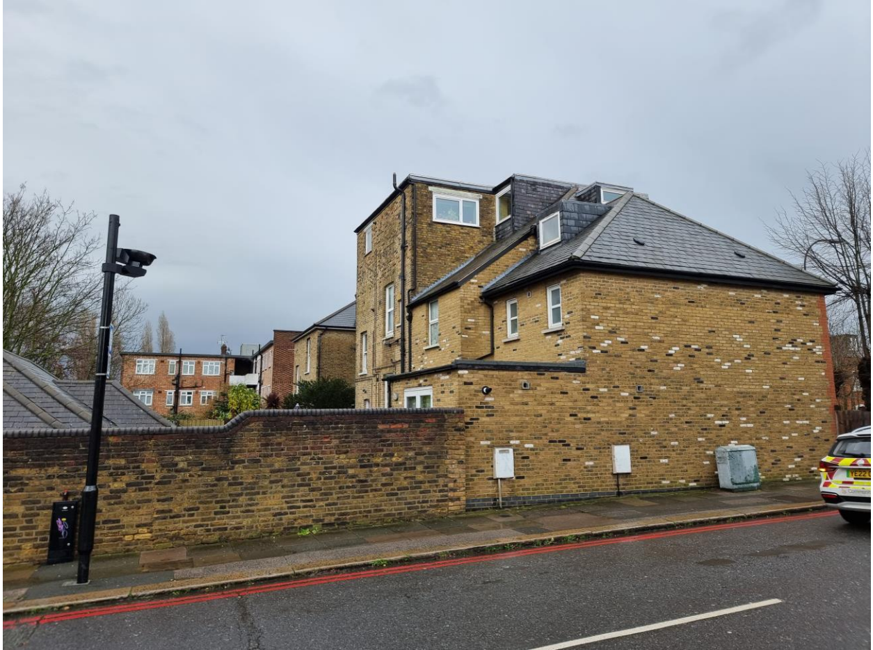
Photo 6 – Rear elevation to No.297
