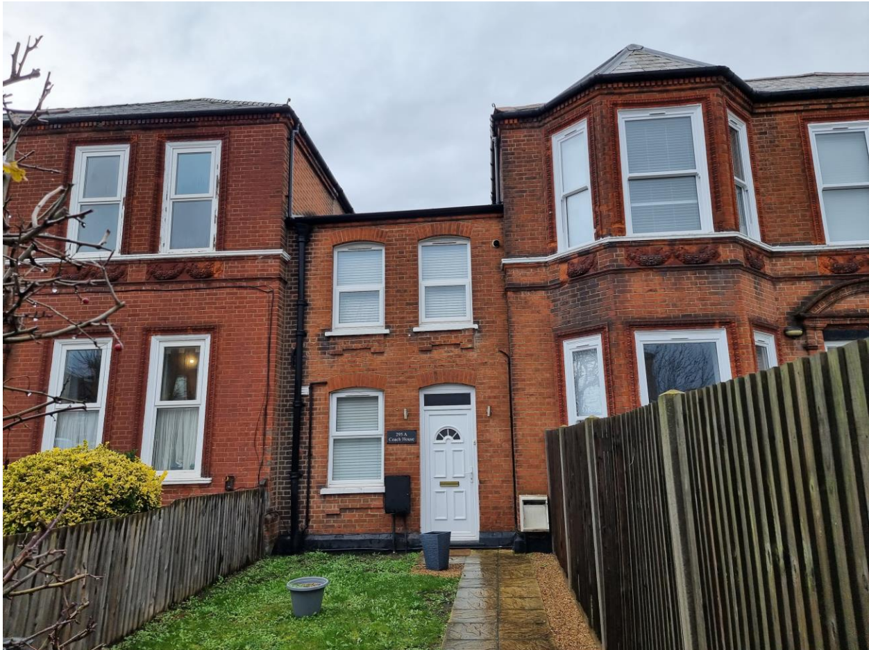
Photo 4 – Elevation showing a coach house between 293 & 295
