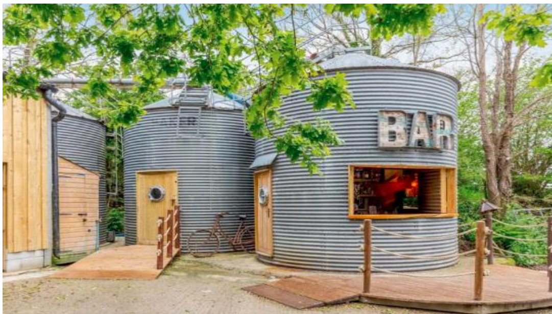
The Bar Silo and Associated facility
