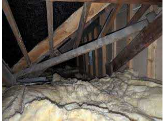
Photo 4. Showing the roof void where it extends over the rear extension
