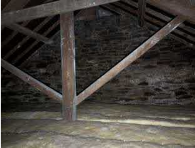
Photo 3. Showing the roof void over the house
