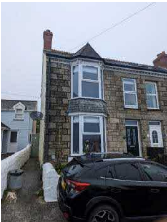
Photo 1. Showing the cottage from the south
