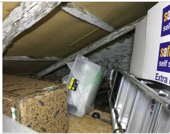
Storage cupboard which forms void over kitchen
