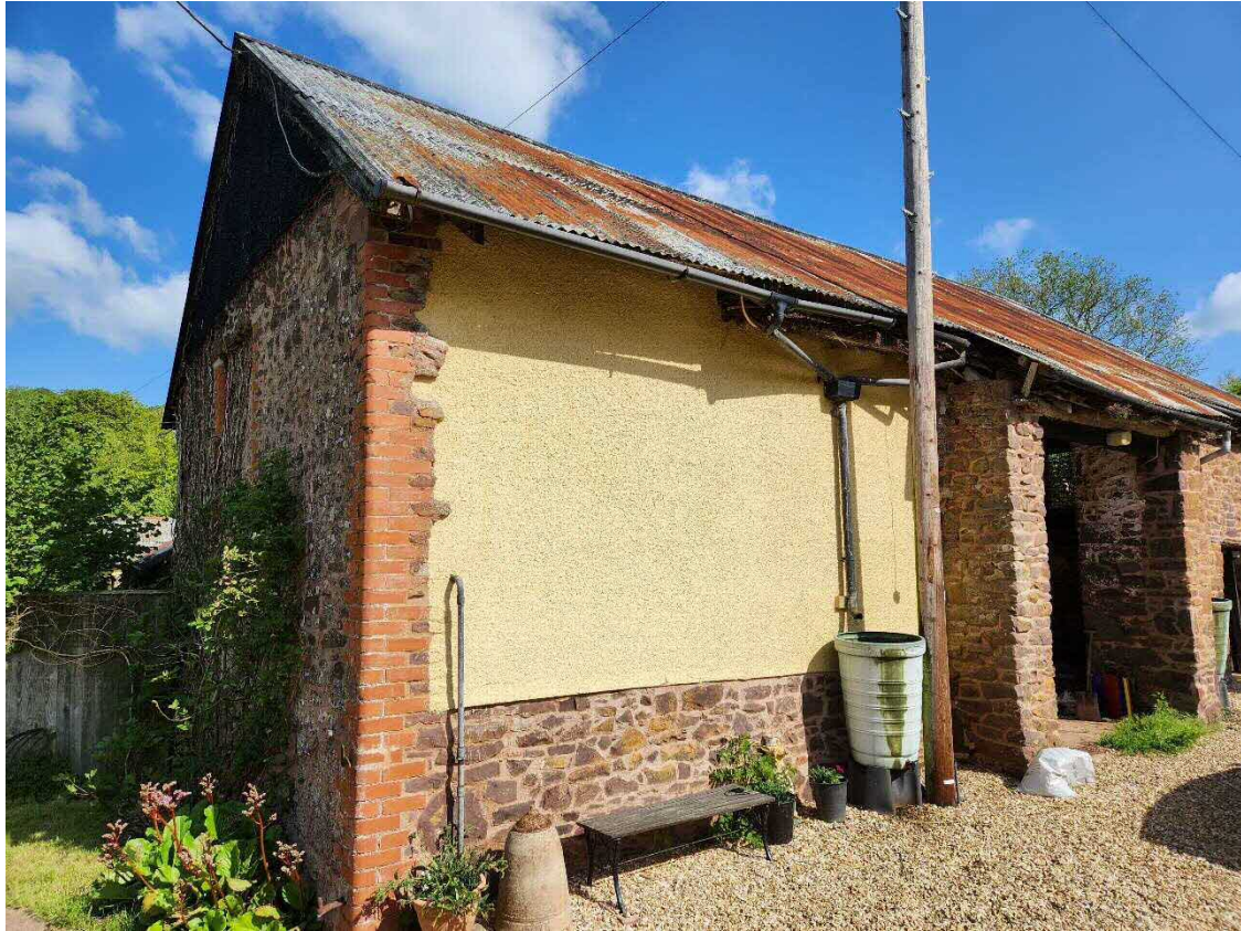
Above: South West Gable/South East elevation of barn
