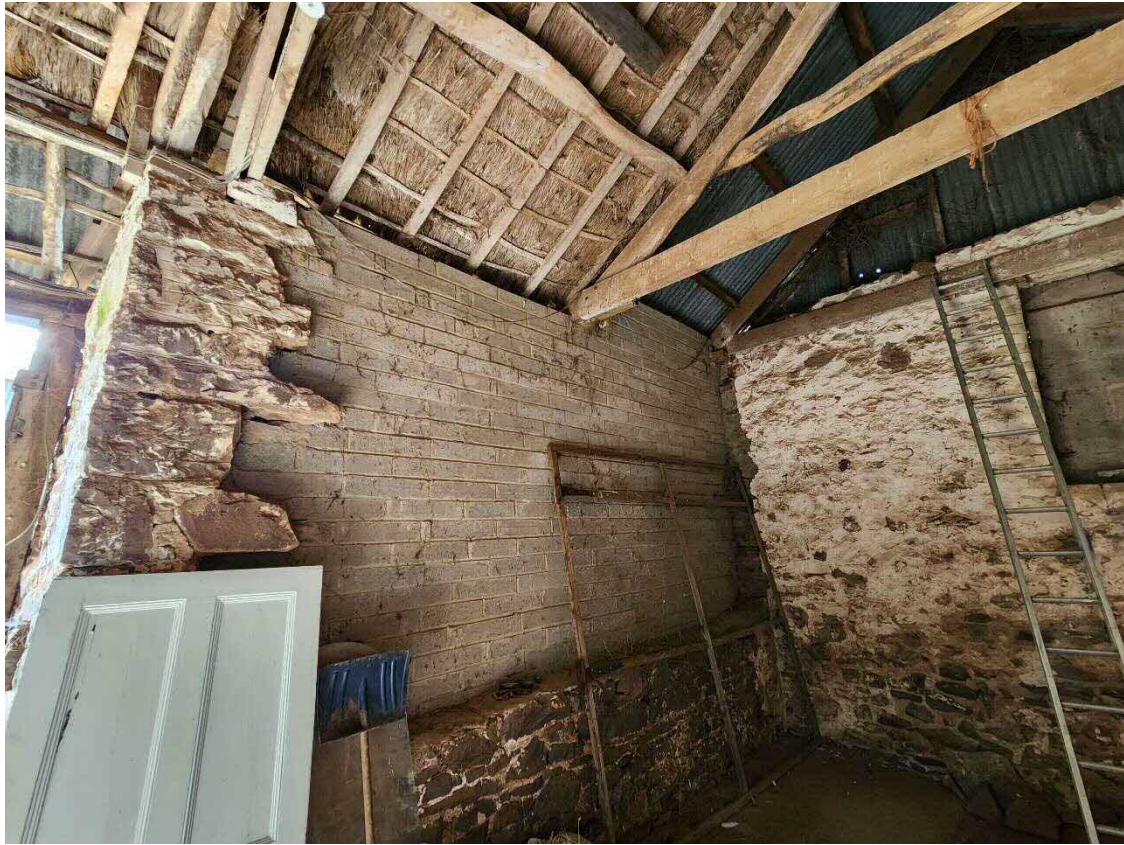
Above: Block on flat infill and stone wall construction internally.
