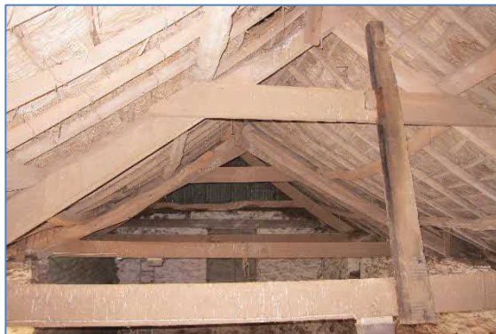
Underside of roof
