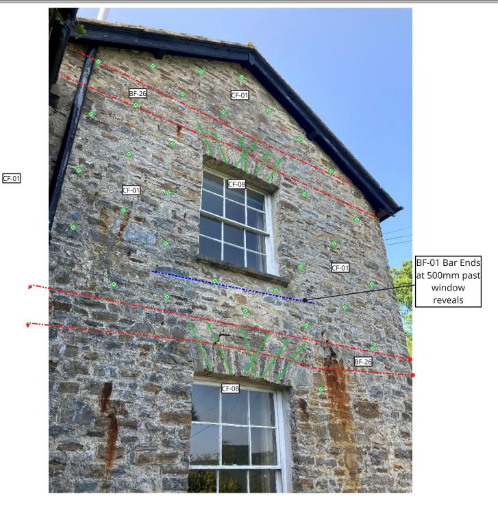
The location, number and length of the fixings, remedial reinforcement and/or Heli Pile® points shown on this drawing are intended only to give an indication of the methods to be used and the amount of material and work that is required to carry out the repairs indicated. The precise number, location and length of fixings may vary depending upon the exact conditions encountered during installation.
