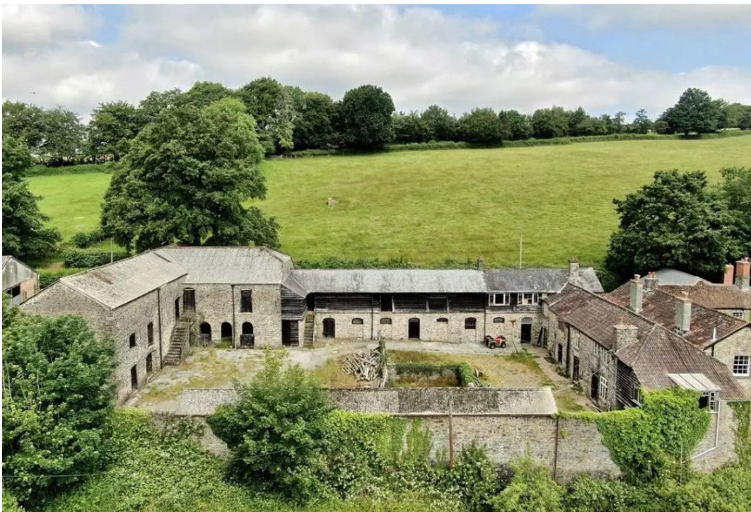
FIGURE 3: DRONE VIEW OF THE LISTED FARMBUILDINGS AND FARMYARD FROM THE SOUTHEAST (©GTH)
