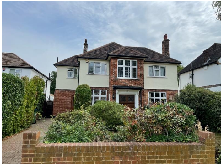
Front and rear views of 59 Guibal Road
