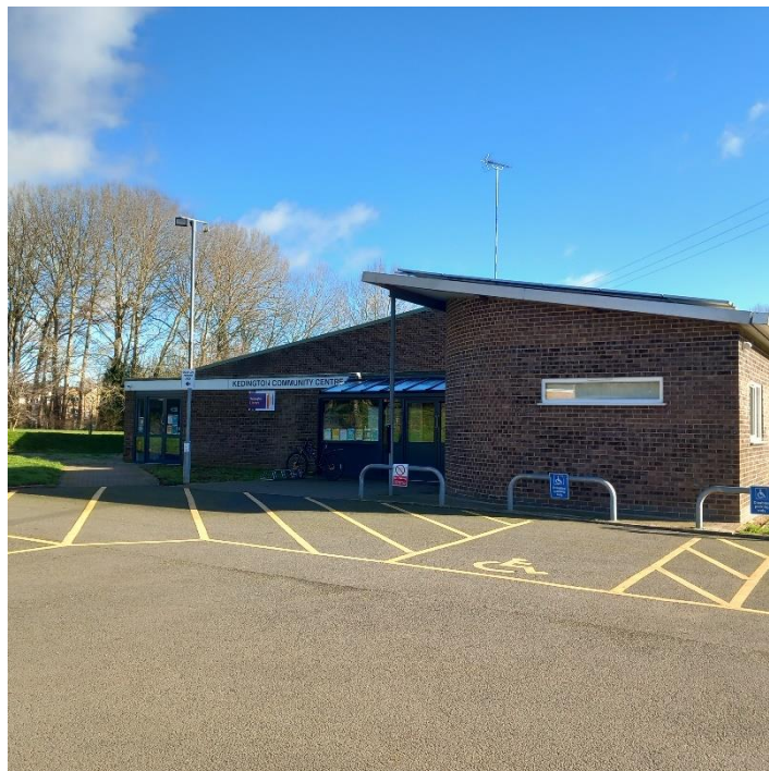
Photograph 1 showing the front (west elevation) of the Community Centre.
