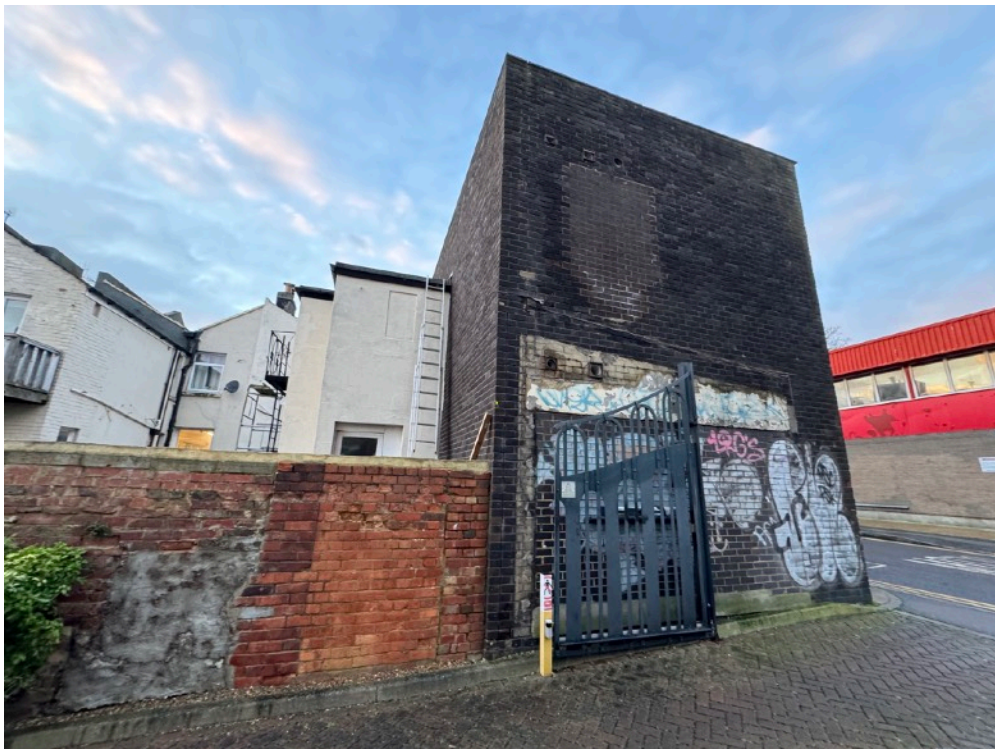
Rear view of boundary wall
