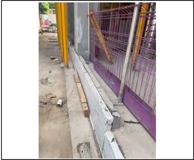
Additional overview of perimeter
