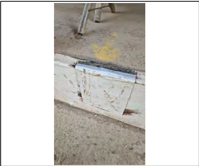
Additional patch repair.
