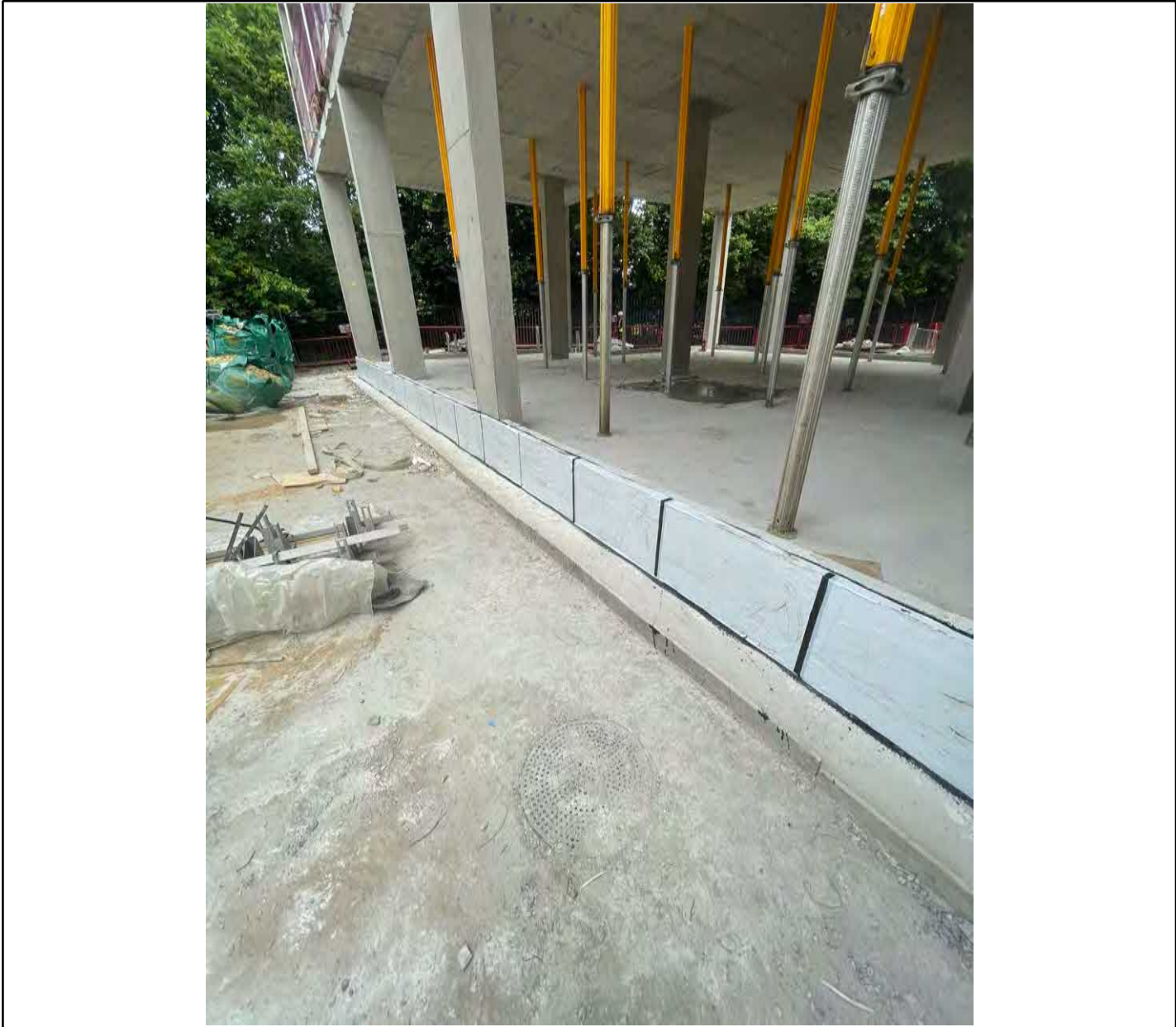
Overview of perimeter termination using Hydroprufe 8000 self adhesive
