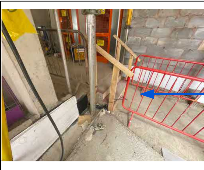
Area behind stairs was not sealed.
