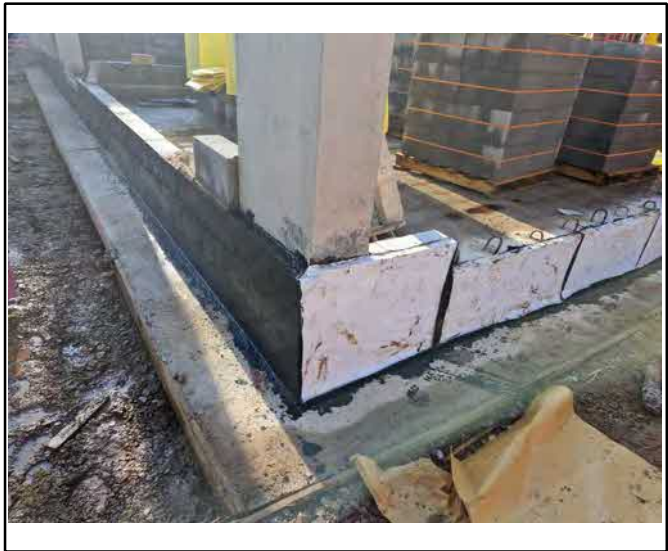
Primer applied prior to Hydroprufe
