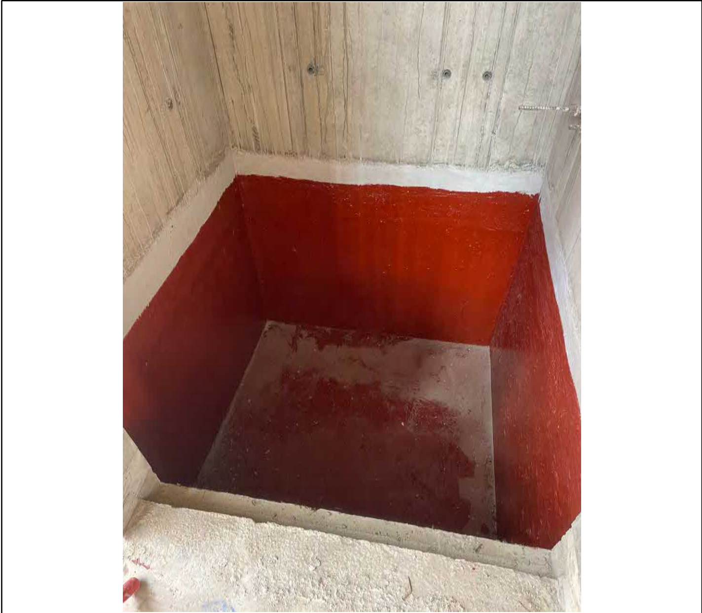
Overview photograph of sealed lift pit using Hydroseal FX and Hydroprufe
