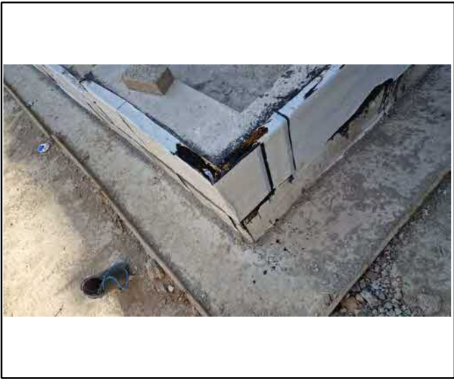
Additional patch repair.
