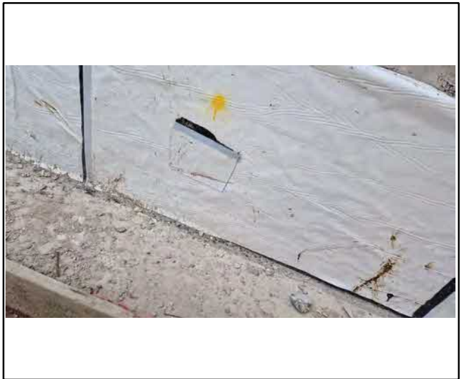
Additional patch repair.
