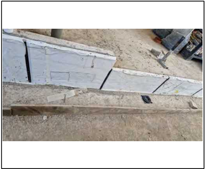
Additional patch repair.
