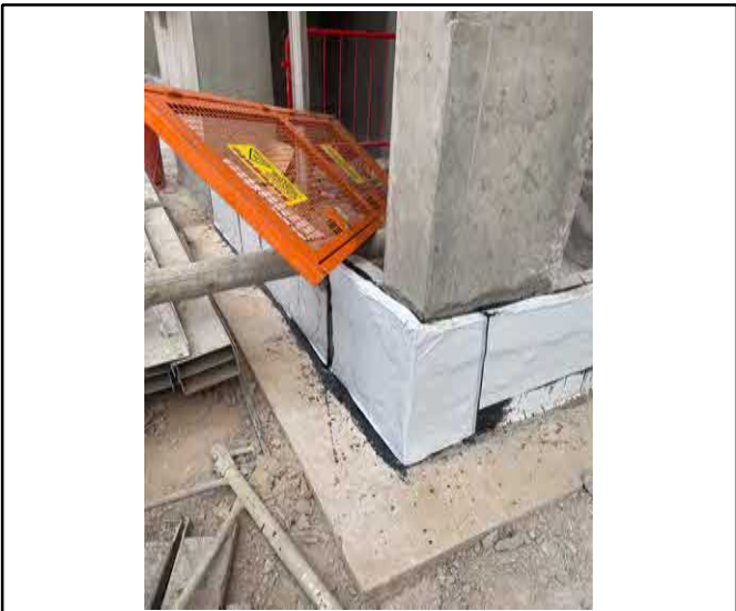
Additional overview of perimeter
