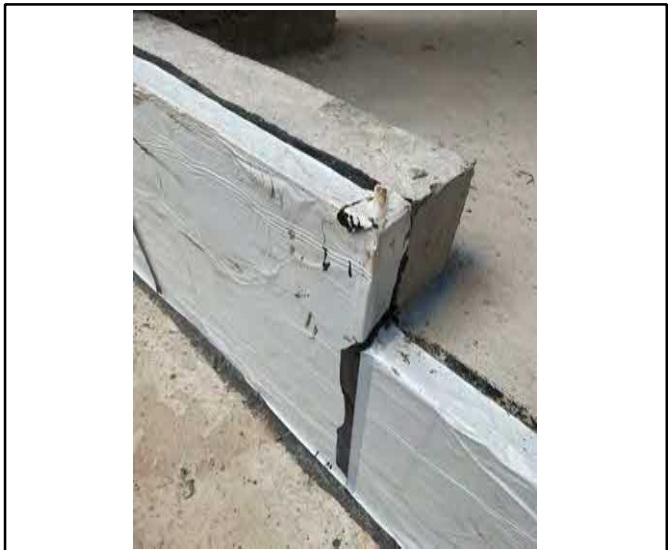
Sealed corner/door threshold.
