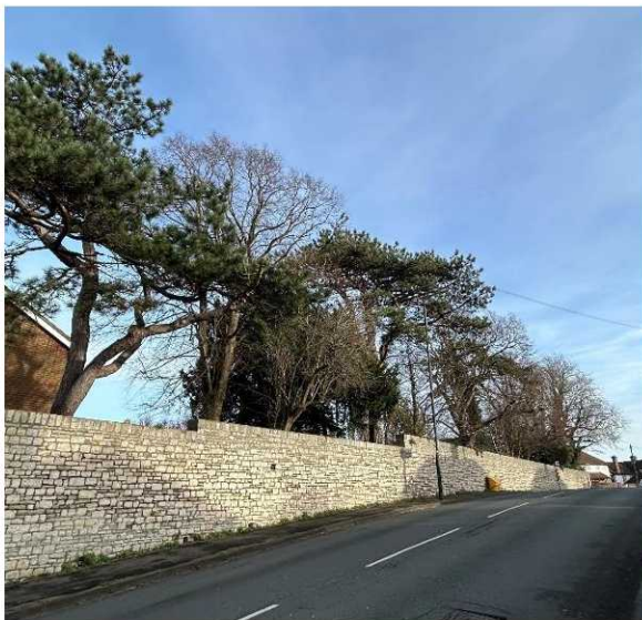
Image 3: Good crown clearance over Redcatch Road.
